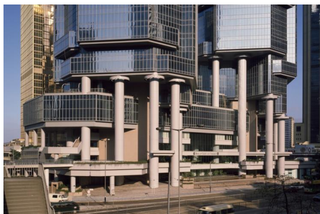
Figure 2-23: Base of Lippo centre
