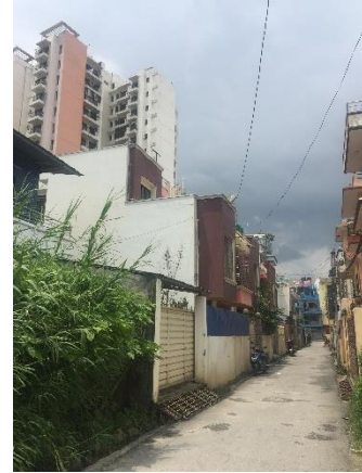
Figure 8-6: showing enclosure of Sun-city apartment
