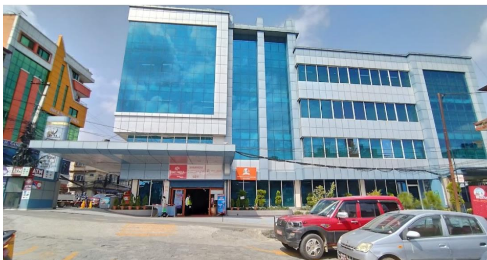
Figure 5-12: View from Surface parking (East side)
