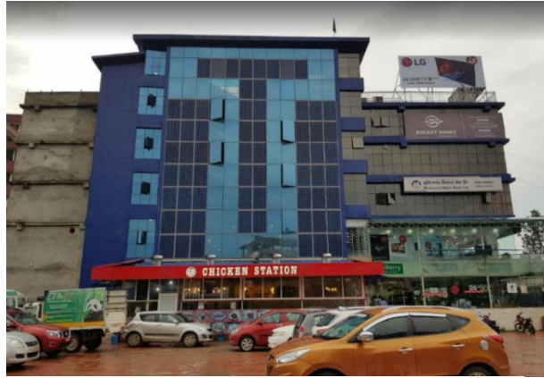
Figure 4-1: Polycrystalline Solar panels used facade of the building
