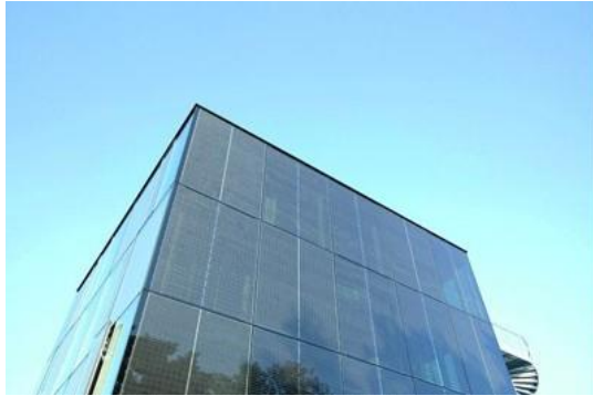
Figure 2-6: Solar PV as facade
