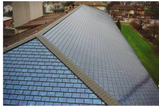
Figure 2-6: Roof Top PV (Lumen Solar)
