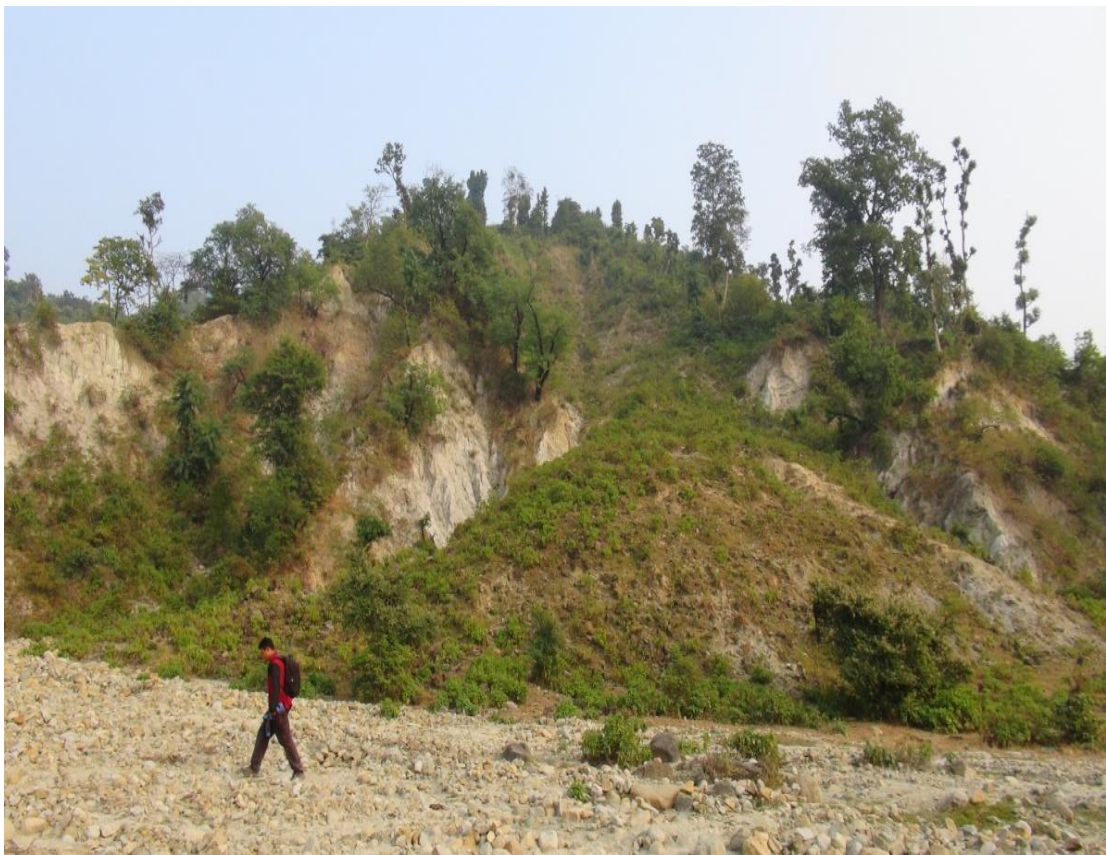
Figure 1 5 Photograph of Simalchaur Landslide
