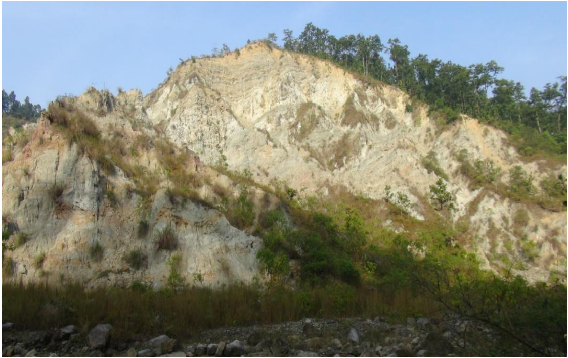
Figure 1.3 Photograph of Setebhir Landslide
