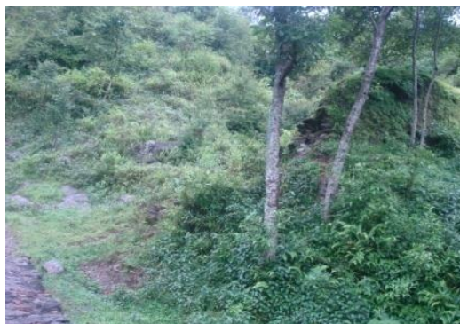
g. Broken wall of the park in Sunkhani VDC
