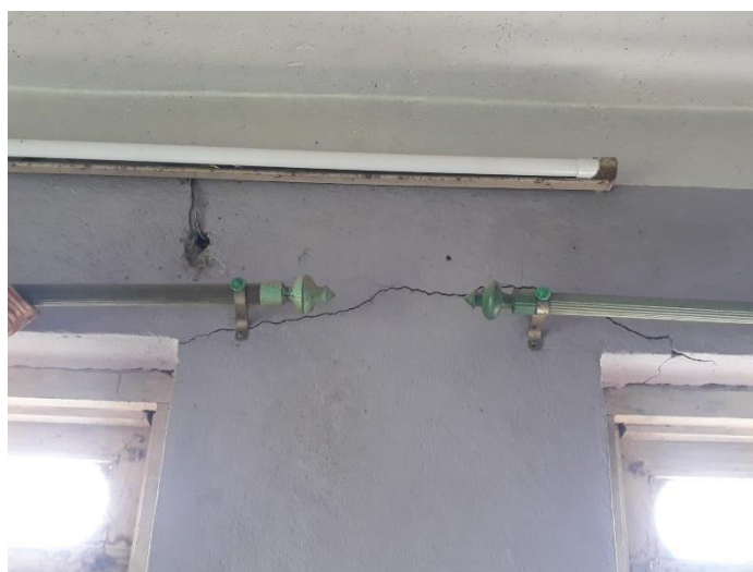
(a) Diagonal Cracks originating from opening
