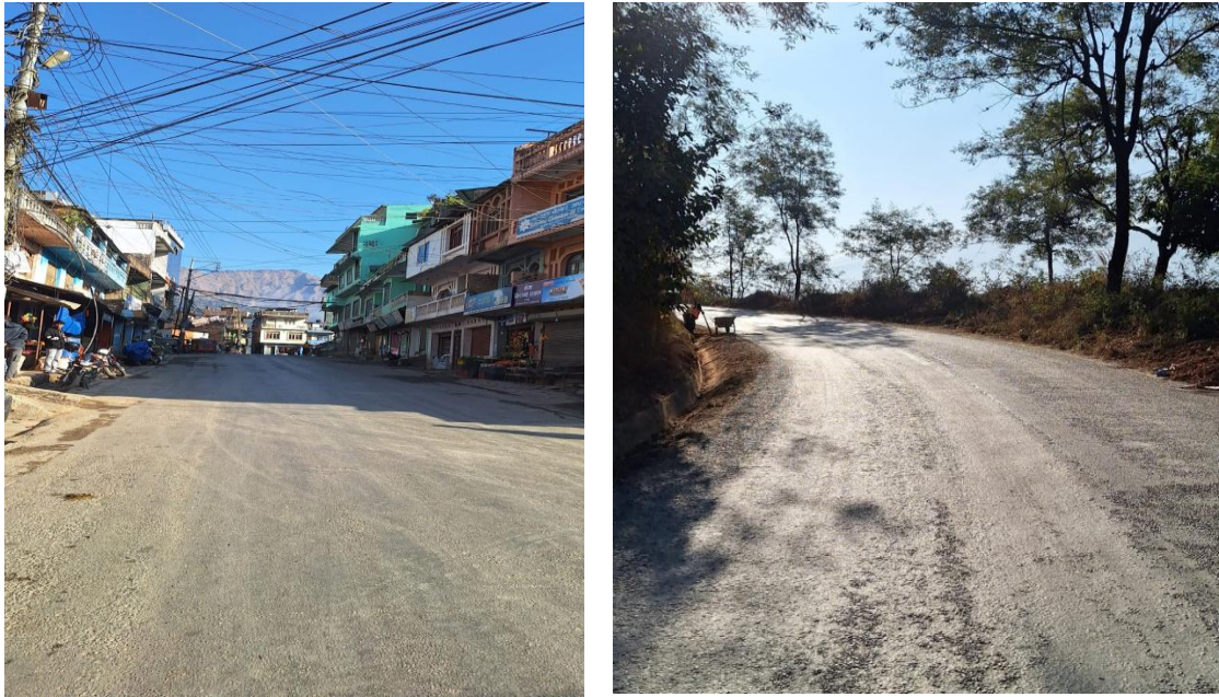
Figure 27 Highway section in Galyang
