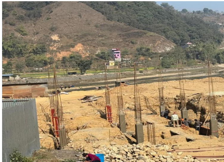
Figure 28 : Ongoing Buspark construction in Waling
