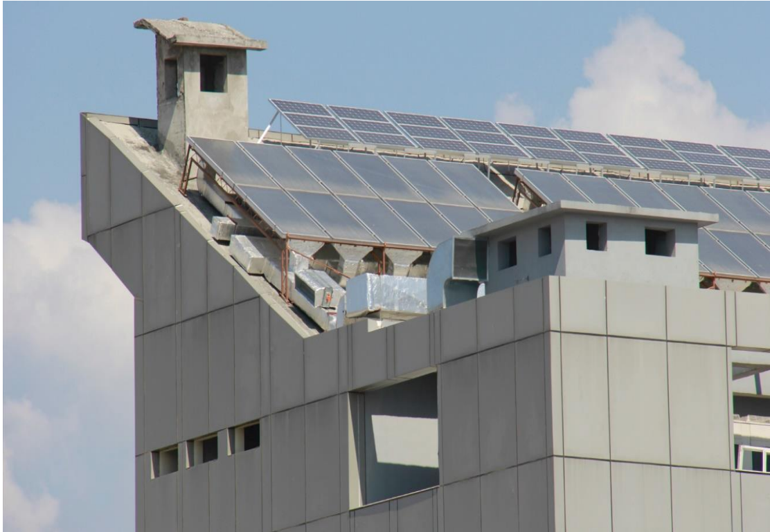
Figure 52: Showing Solar Panel Placed on the Terrace (Source: archinect.com)
