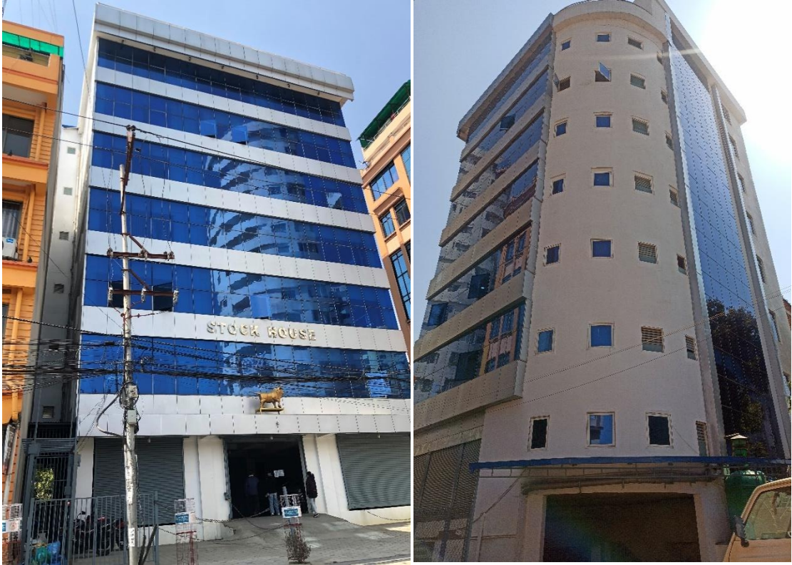
Figure 65: Building Facades- Stock House
