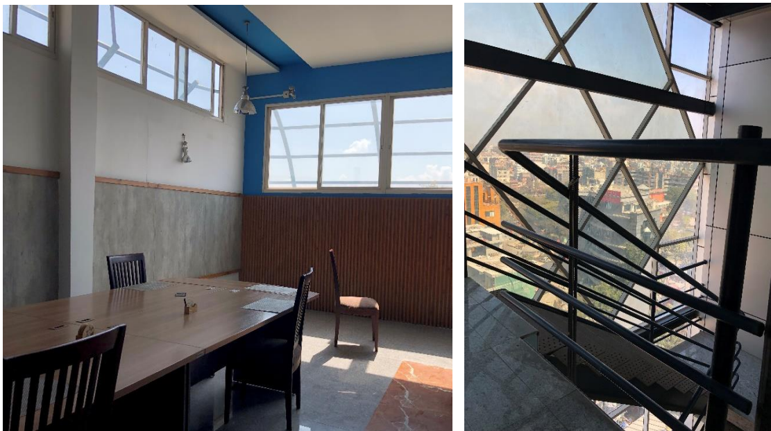
Figure 31: Daylight at Meeting Hall and Staircase areas
