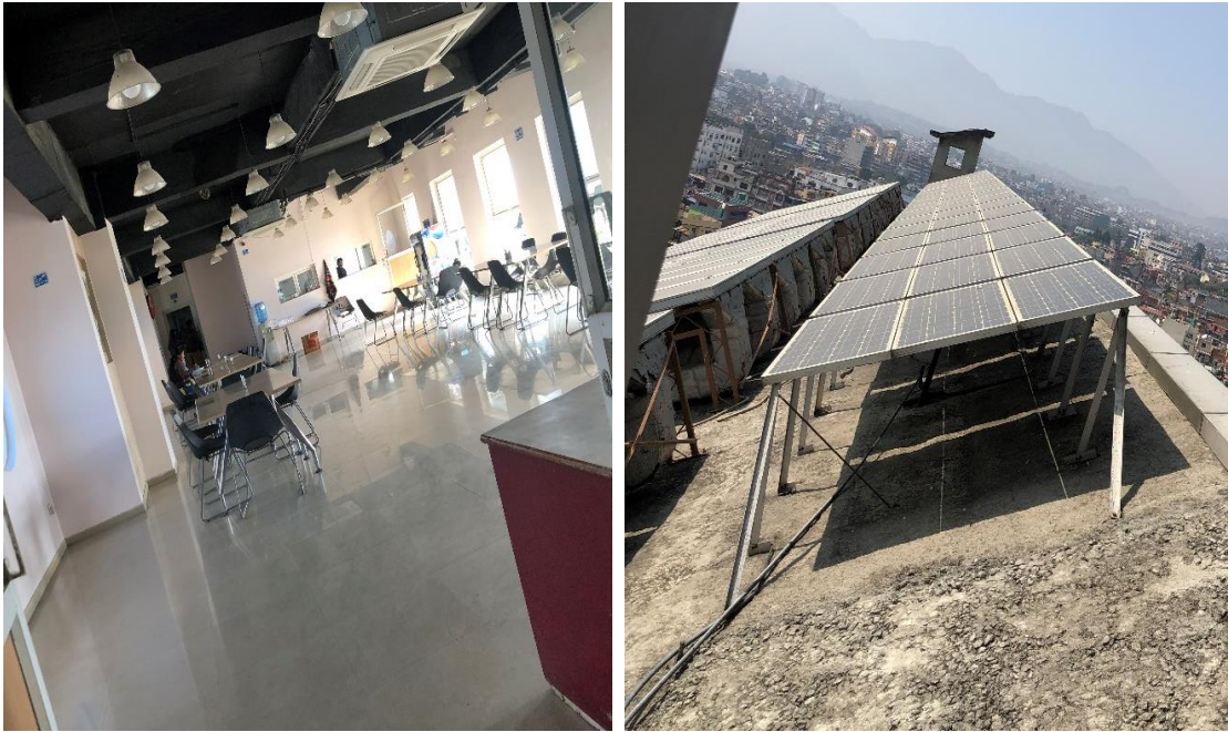
Figure 61: Roof Top Cafe and Photovoltaic Cells- BPC
