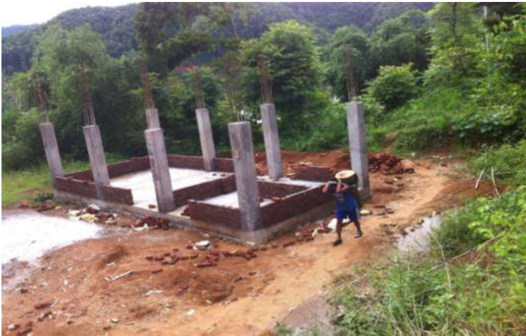
Construction site of Bote Museum
