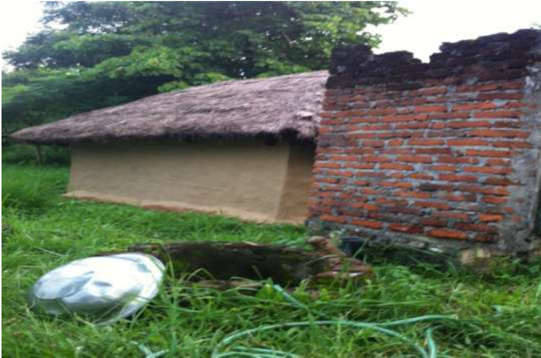
Bio-Gas plant in Bote community
