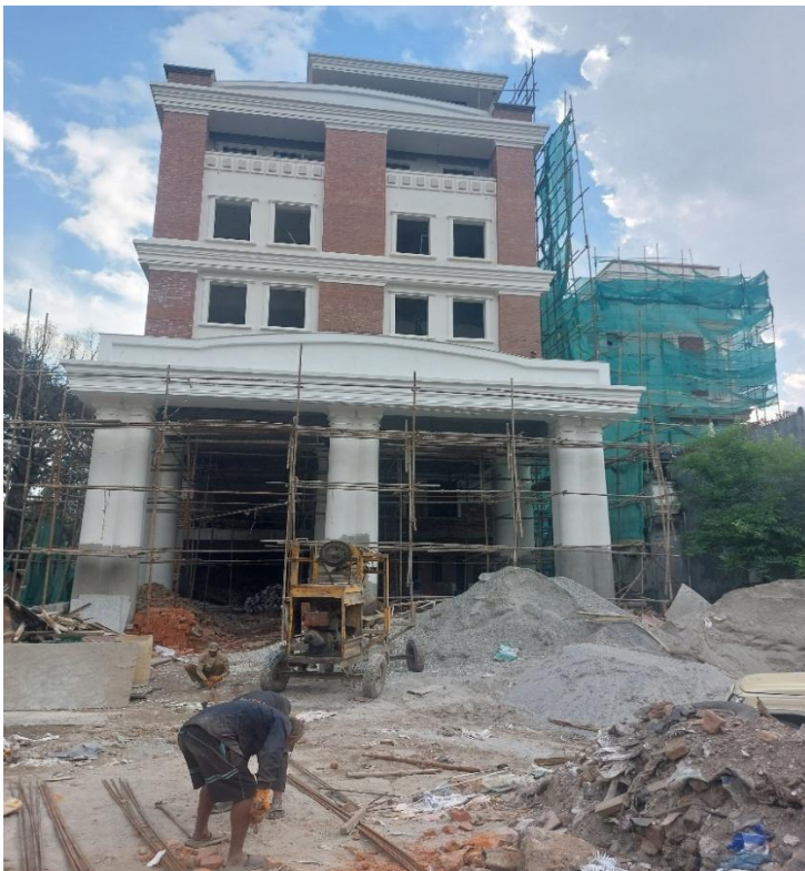
Project B (Integrated Hulak Office Building, Babarmahal, Kathmandu)
