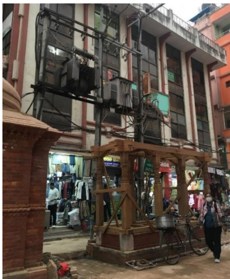
Figure 71: Construction of Pati in Bhotahity
