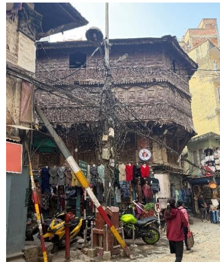
Figure 80: Vacant house in Balkumari road
