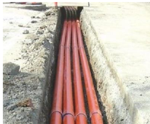
Figure 85: Installation of underground power cables
