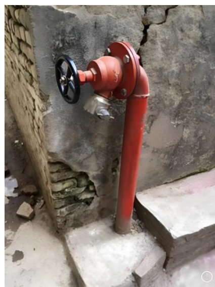
Figure 70: Installation of Fire Hydrant
