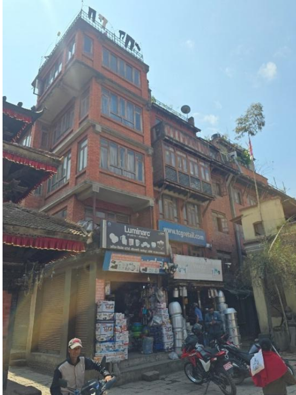
Picture 3 Least compliant buildings - BKT-09, Golmadi, Bhaktapur
