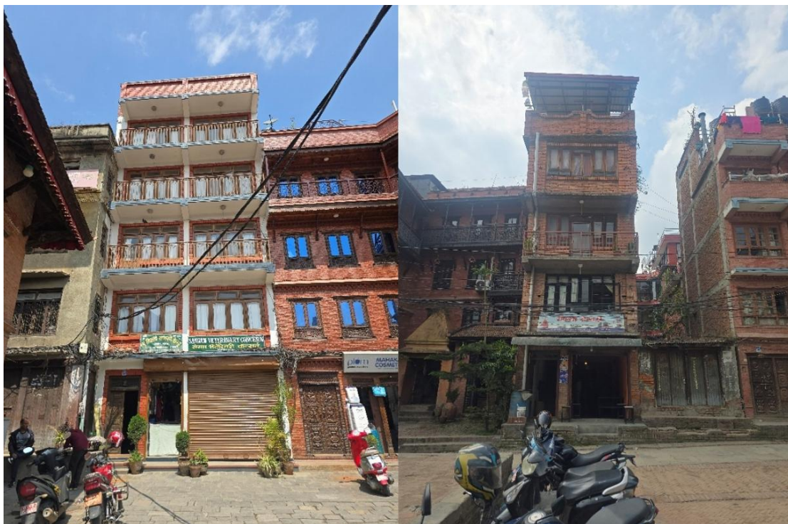
Picture 5 Examples of Non-compliance (rolling shutter violations)
