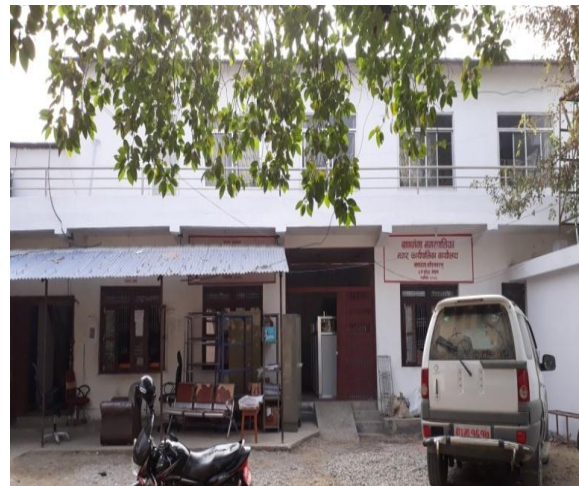
Figure 8: Office Building of Municipality
