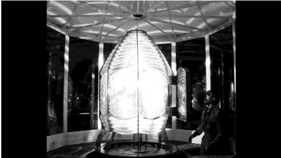
Figure 17. The egg-shaped structure which houses circular Fresnel lens [source: screenshot of The Lighthouse 01:43:43]
