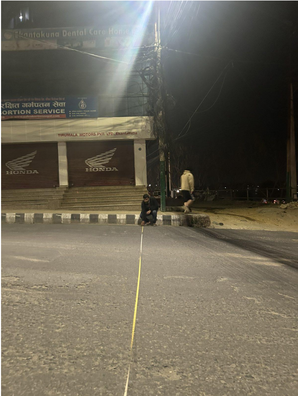
Tape Measurement for Existing Geometry
