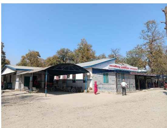
Madhyabindu Hospital Before
