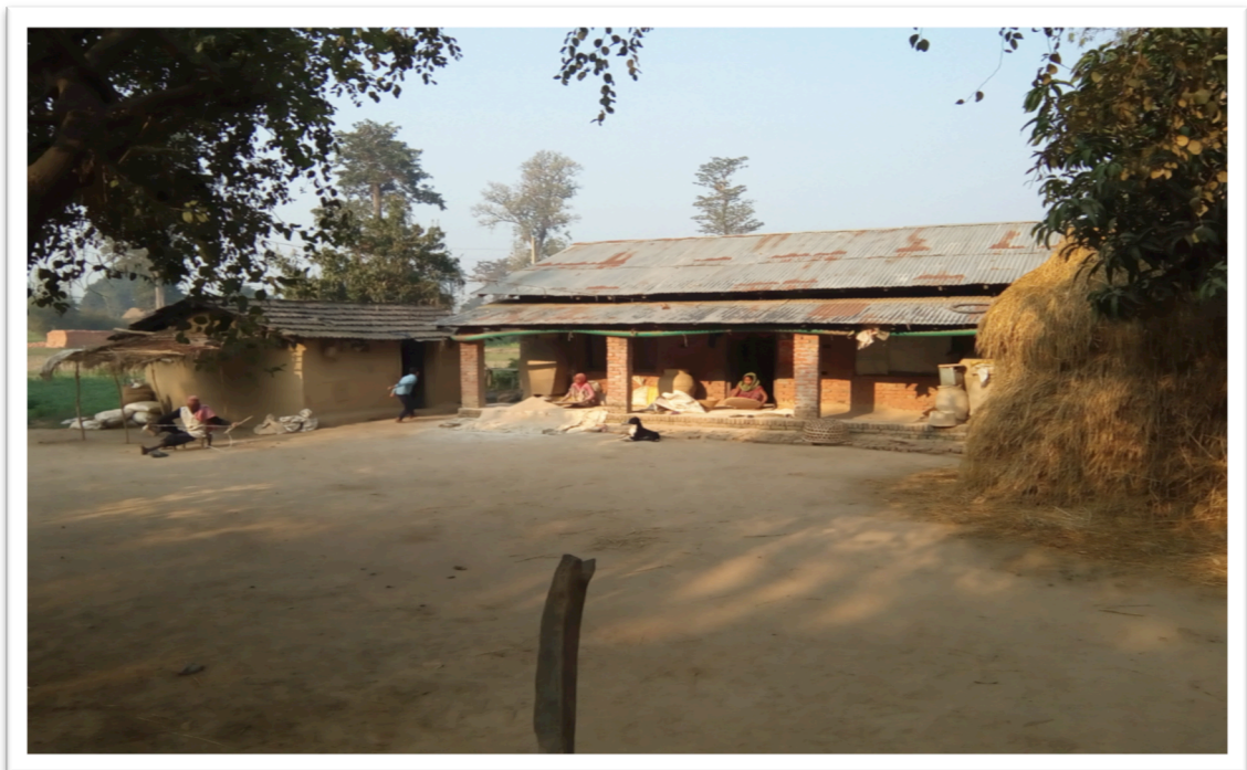
Picture No. 2 Traditional Shelter of Kamaiya community
