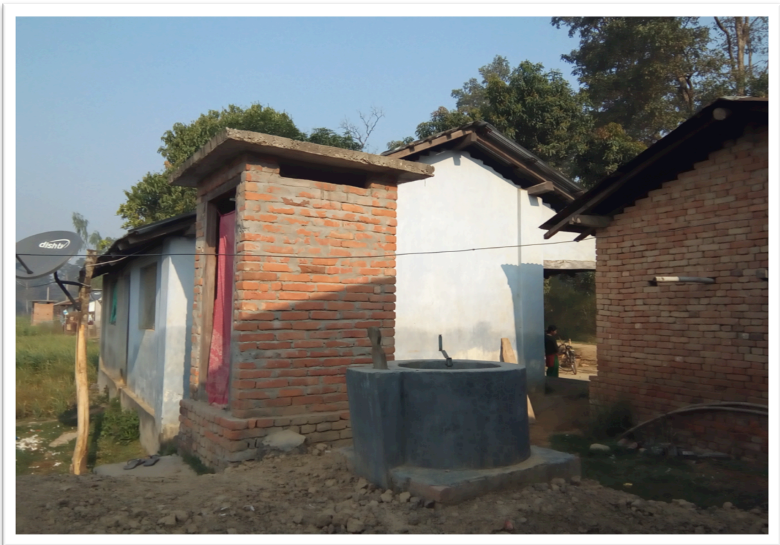
Picture No. 6 Toilets attached with Bio gas plant
