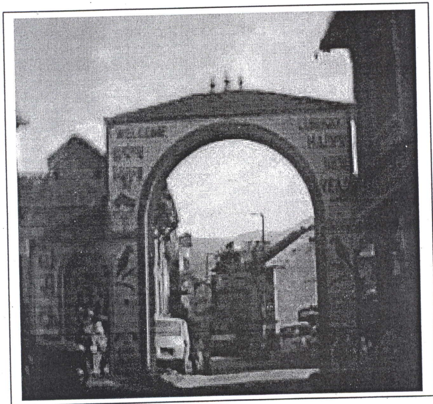
Plate 3.1: Entrance Gate of Core Area of Lubhu
