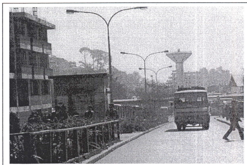
Plate 5.5: New Bus Park after the Construction of Ring Road
