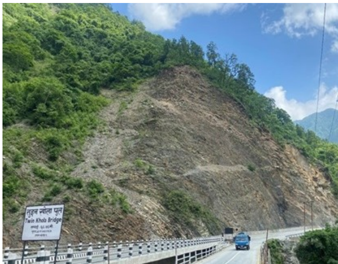
Figure 1: Twin khola Area (CH 33+900) Before massive landslide
