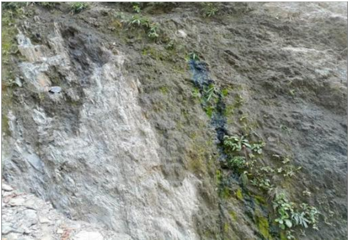
Figure 4-4: Exposure of rock mass at L2.
