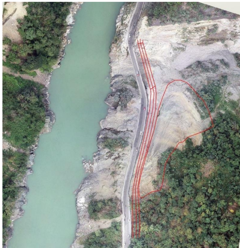
Figure 1-3: failure plane and geometry of the landslide.
