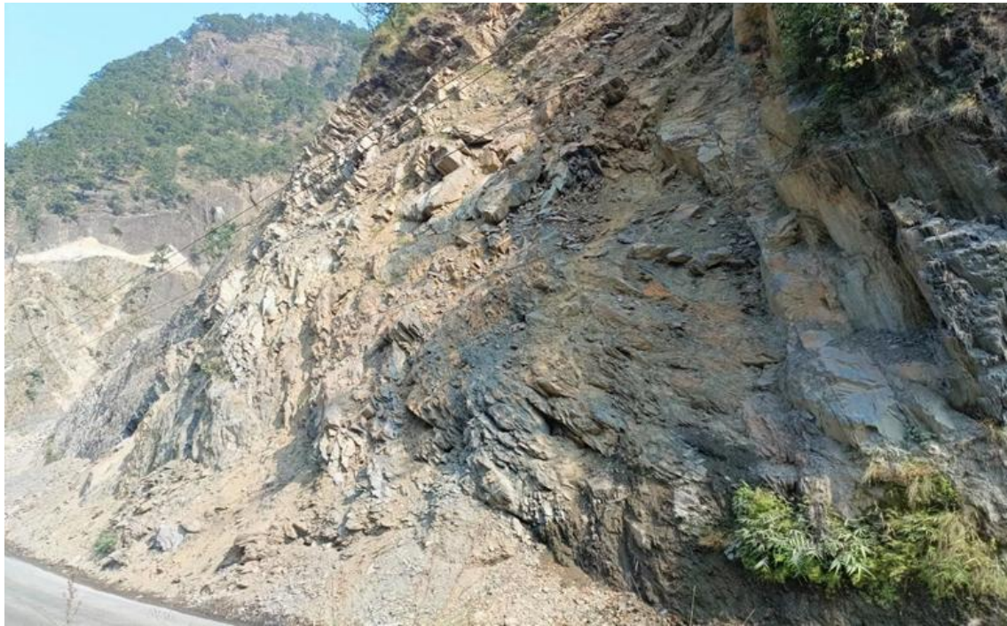
Figure 4-7: Exposure of rock mass at L5.
