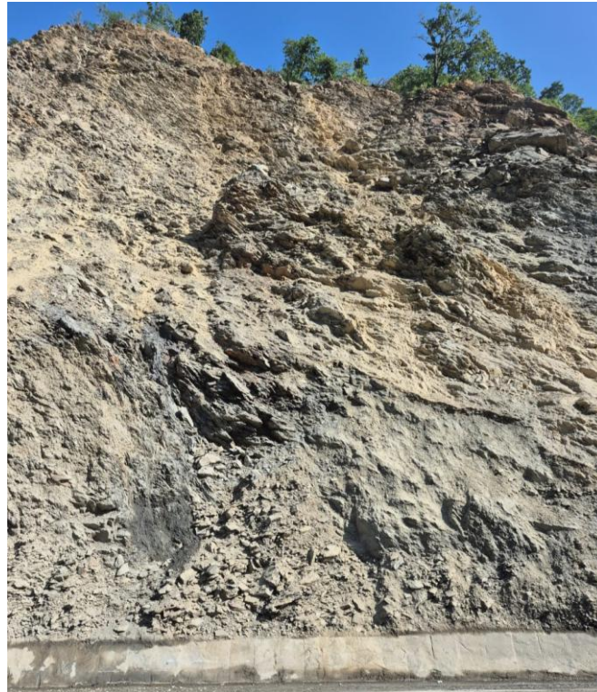
Figure 1-5: View of slope material of roadside cut slope.
