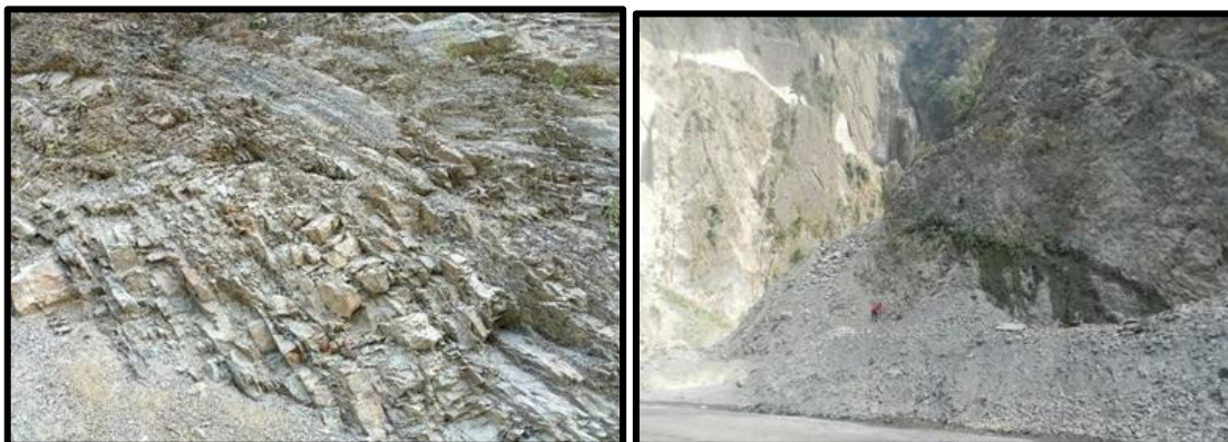
Figure 4-3: Exposure of rock mass at L1.
