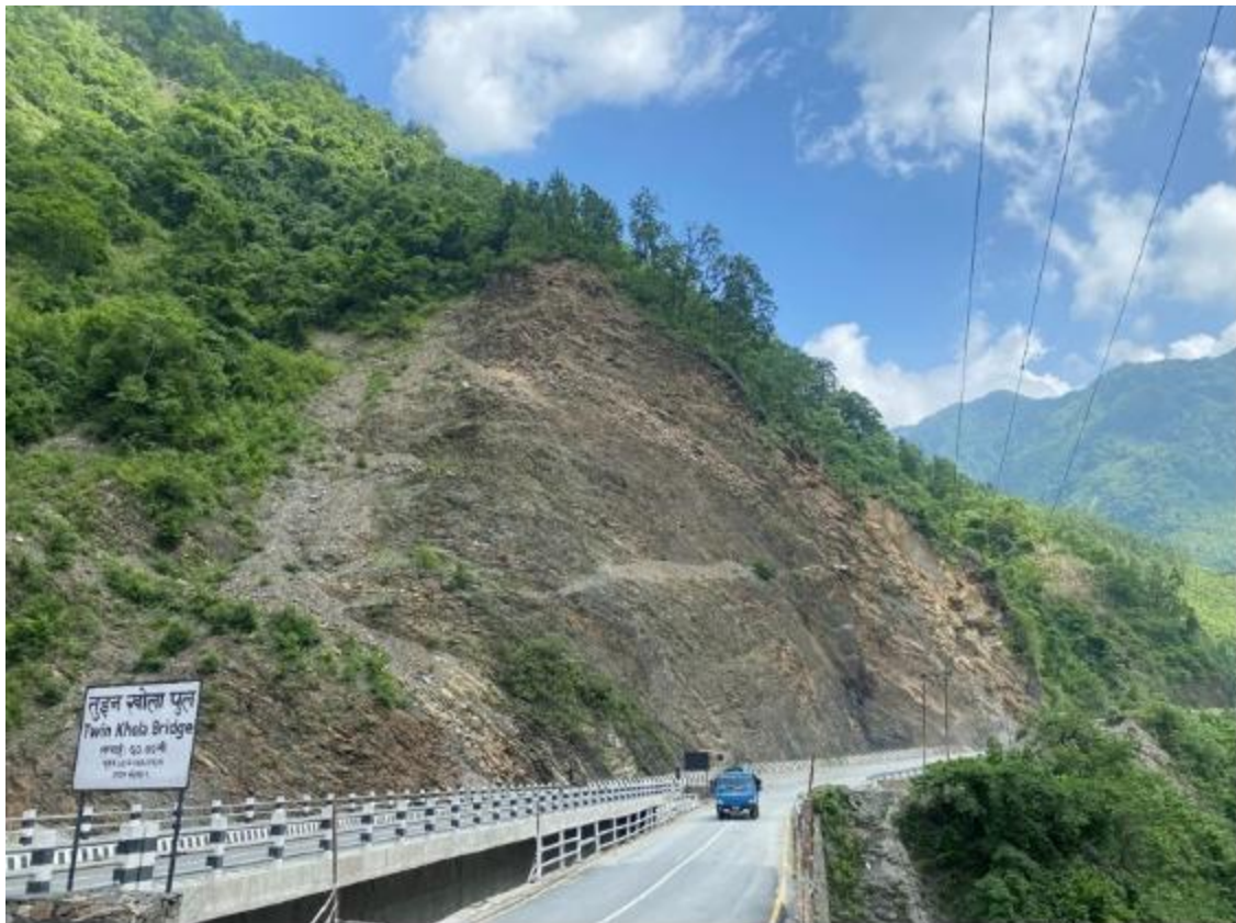
Figure 3-1: Tuin khola area (CH 33+900), before massive landslide.
