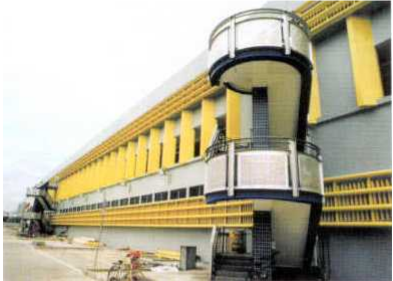
Figure 109: Acoustic louvres for noise mitigation
