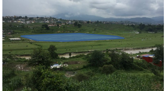
Figure 125: Site View from Dakshinkali Road
