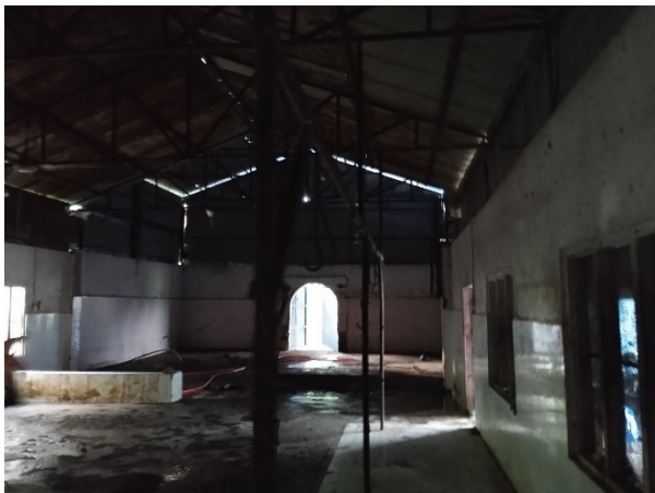
Figure 78: Interior of Slaughter hall
