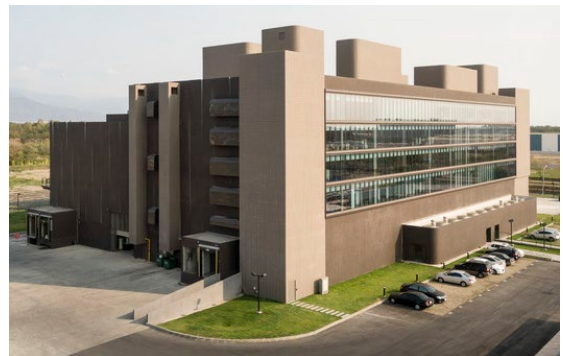
Figure 121: View Showing Uneven Heights of Lift
