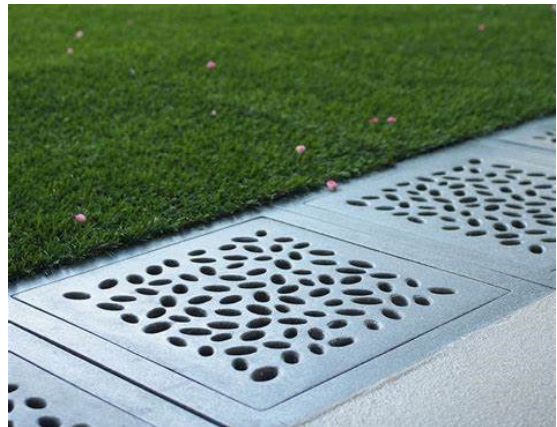
Figure 157: Stone Trench Grates
