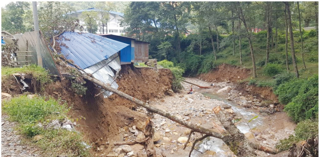
Destruction of the Godawari River, the source of Iku-dha Irrigation Canal, due to the recent catastrophic rainfall of September, 2024
