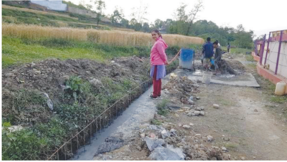
Observing the maintenance of the canal
