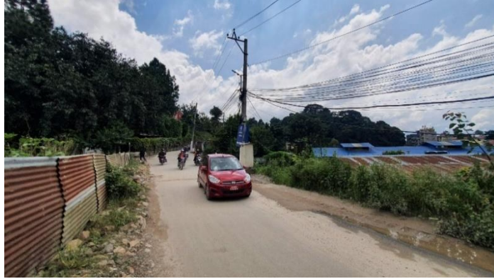
Figure 133: Electrical Distribution for the Site
