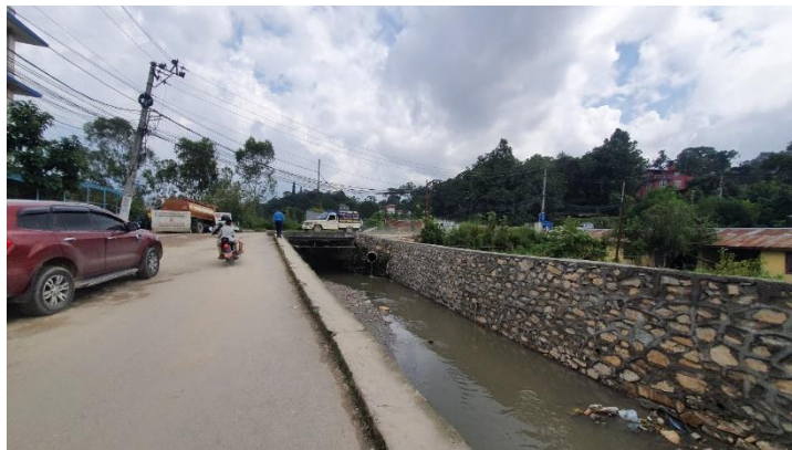
Figure 134: Drainage in the Samakhusi River
