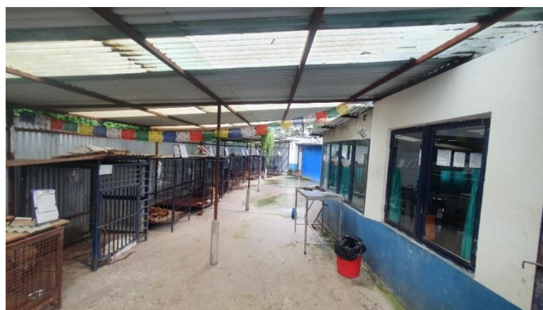
Figure 67: KAT Center Roofing System
