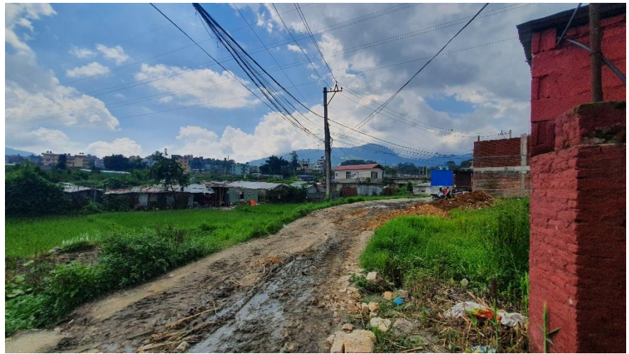
Figure 72: Access Road Leading to the Facility
