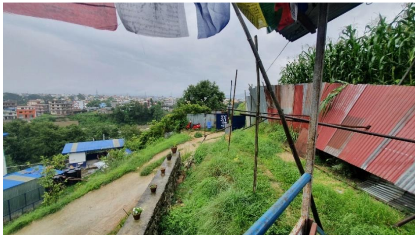
Figure 69: Temporary CGI Fencing in KAT
