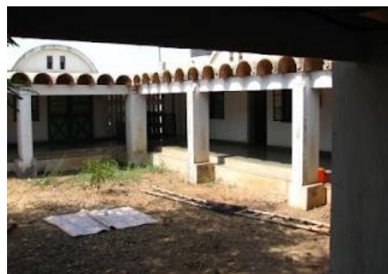
Figure 126: Concrete Roof Vaults
