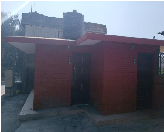
Figure 19 Public toilet in locked state in midday
