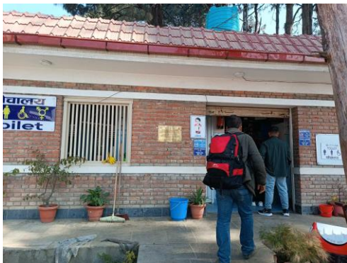
Figure 15 Public Toilet in Swoyambhu
