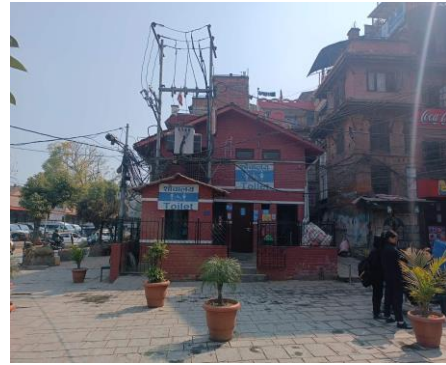
Figure 8 Public Toilet in Mangalbazar
