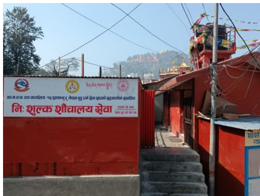
Figure 11 Public Toilets upstairs
