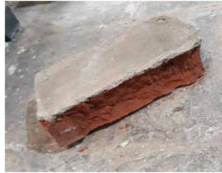
Figure 31 Failure of sample along face
