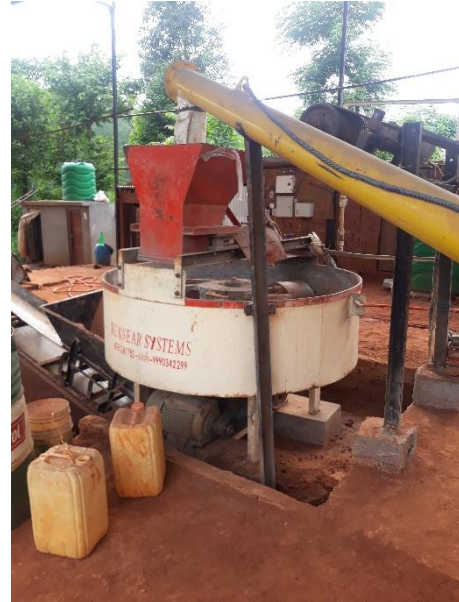
(b) Mixing soil, cement, and additives
