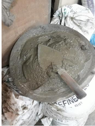
(a) Mortar preparation
