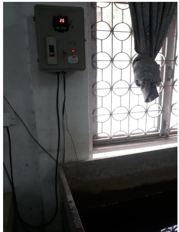
Figure 25 Curing tank with controlled temperature
