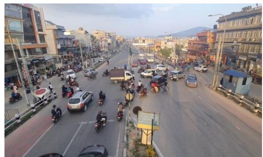
No proper intersection layout at Kaushaltar
