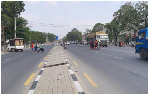
No central dividers & pedestrian crossing marking at Thasikhel
