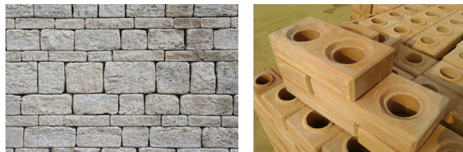
Figure 3: I-Stone and II-CSEB as Wall Construction Materials
