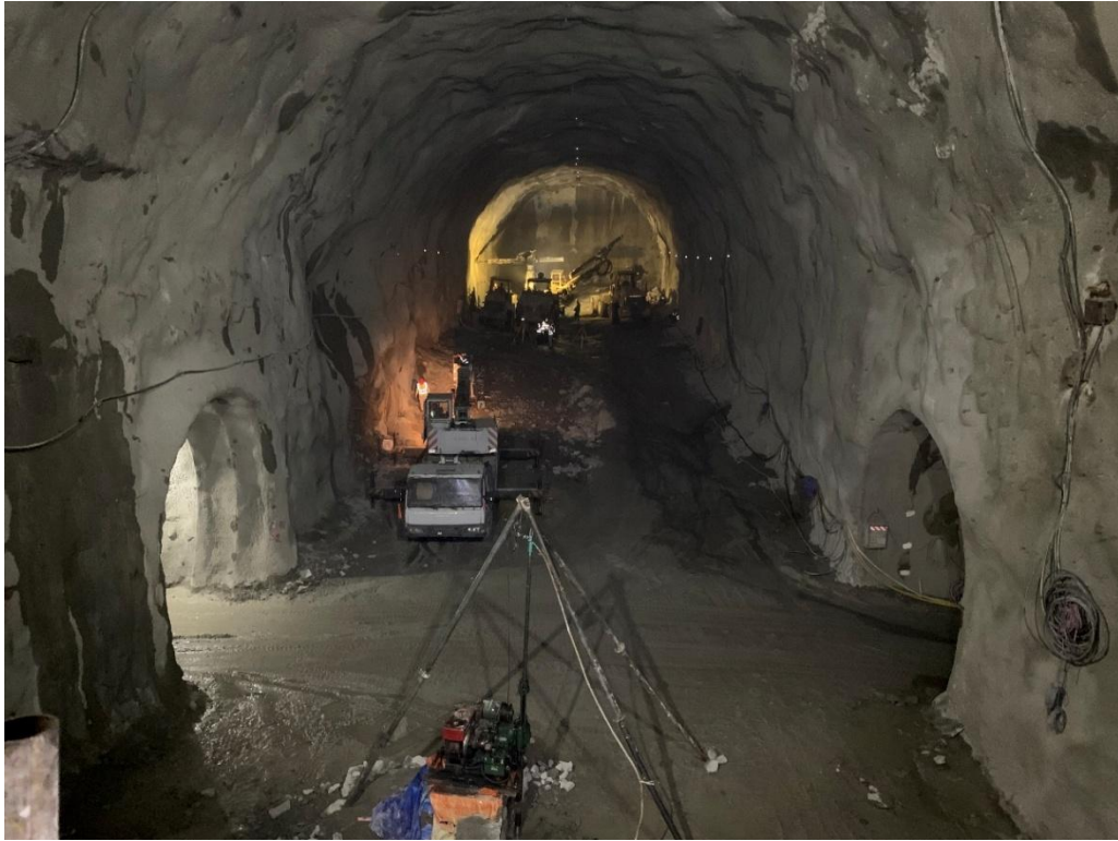
Figure 7-0.1: Excavated powerhouse cavern (crown and first bench)
