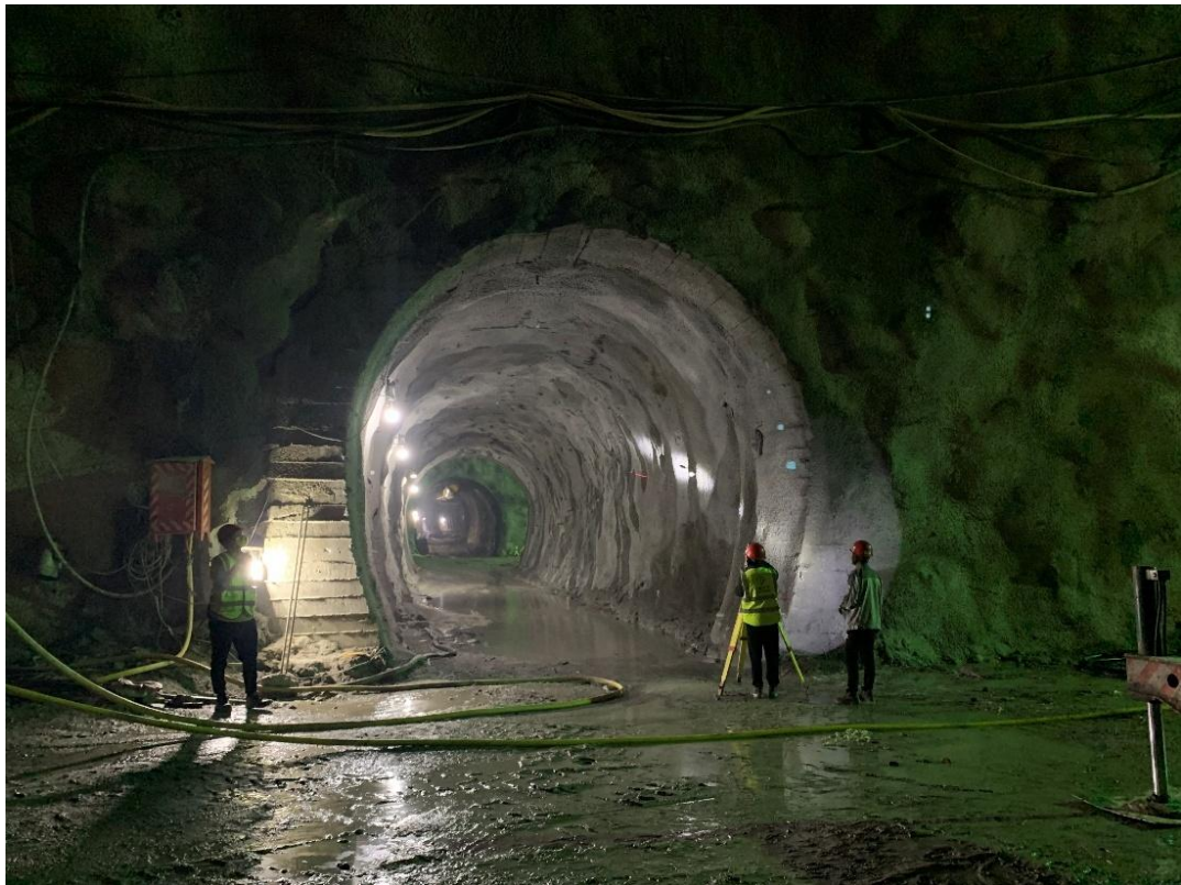
Figure 7-0.5: Tunnel connecting powerhouse and transformer cavern
