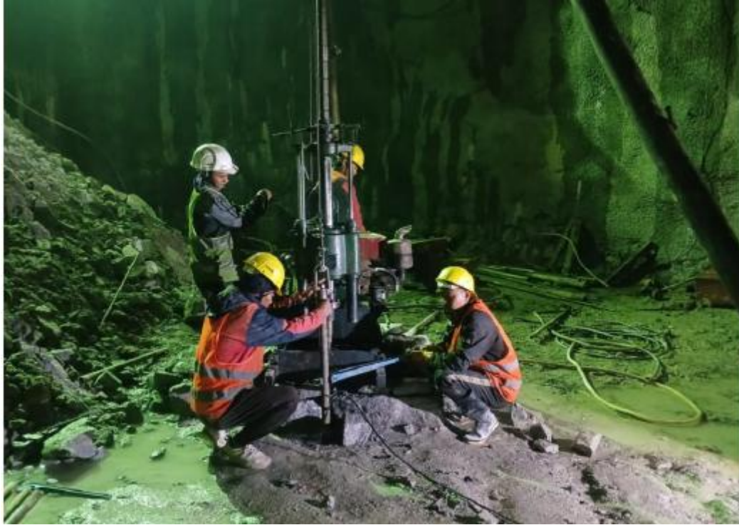
Figure 4.2: Drilling at powerhouse cavern
