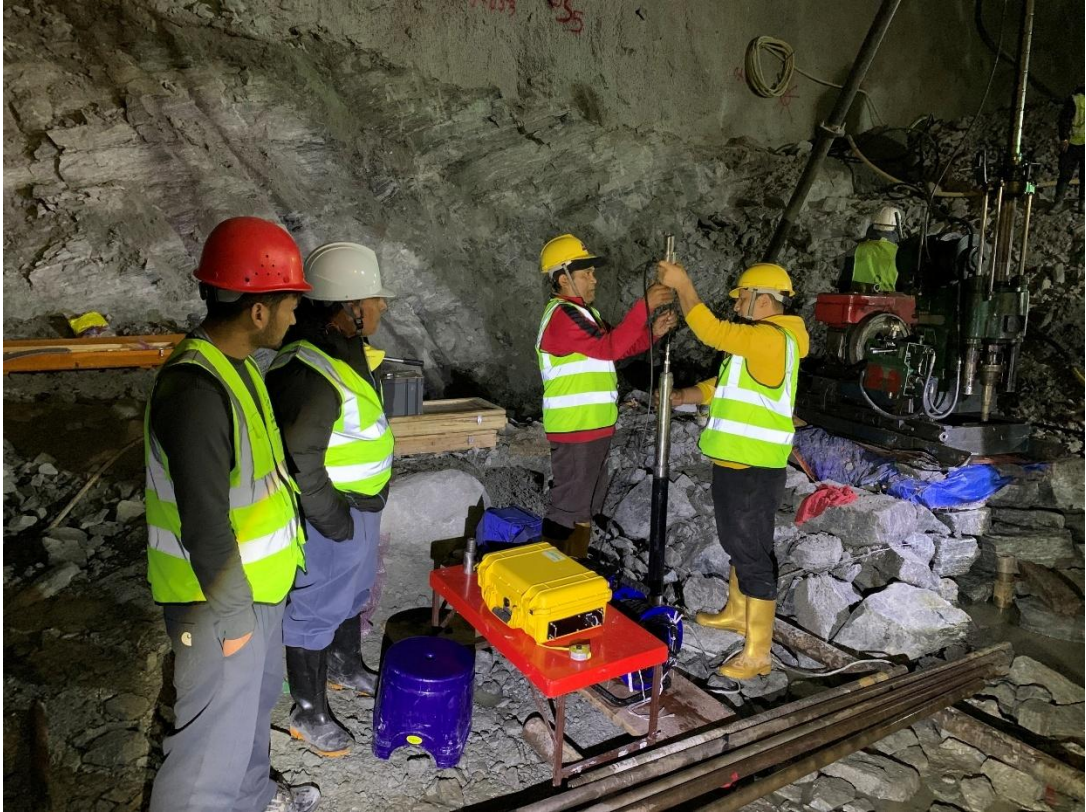
Figure 7-0.4: Preparation of pressuremeter test at powerhouse cavern
