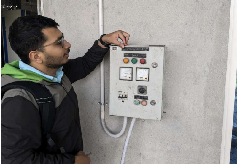
Figure 42:Panel Installed for Boring pump
