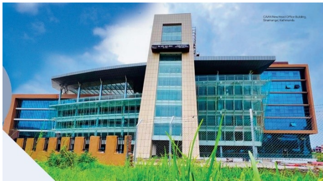
Figure 2: New CAAN Head Office Building at Sinamangal
