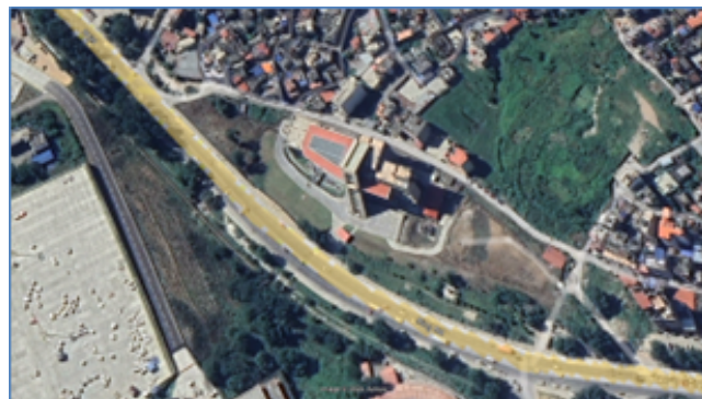
Figure 1: Aerial view of CAAN Building @source : Google Earth
