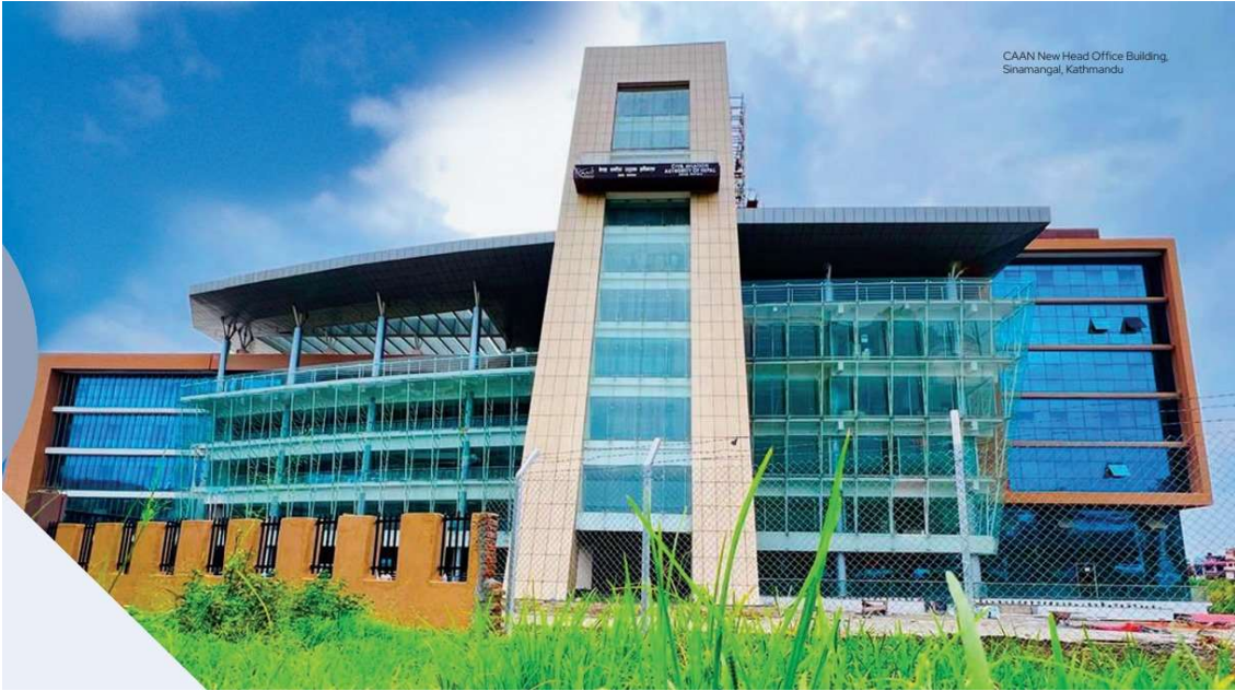
Figure 2:CAAN New head office Building, Sinamangal (Source CAAN Report)
