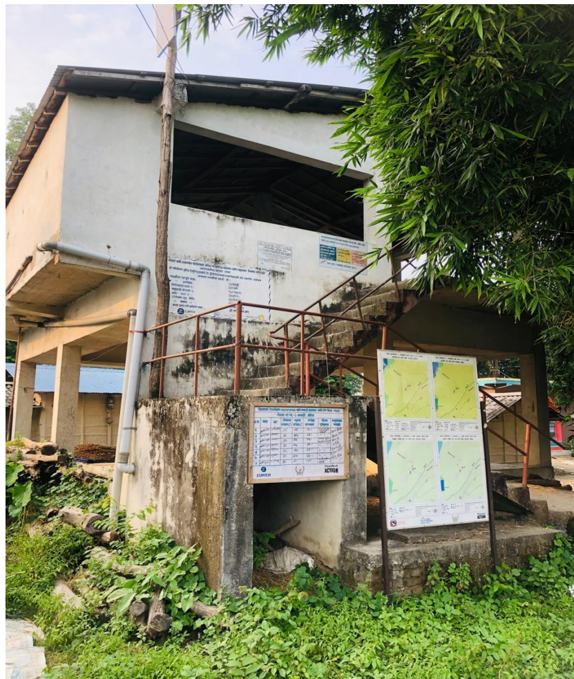
Shelter house of Geruwa-3
