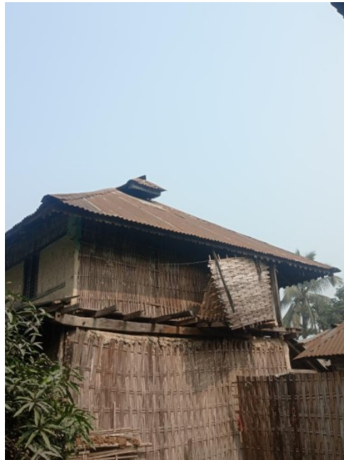
Figure 4: Case study building
