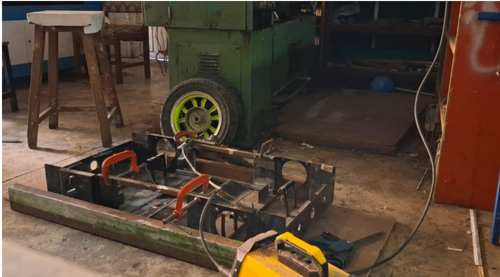
Figure 3: Preparing the Jig Fixture for the Assembly Setup Prior to Welding
