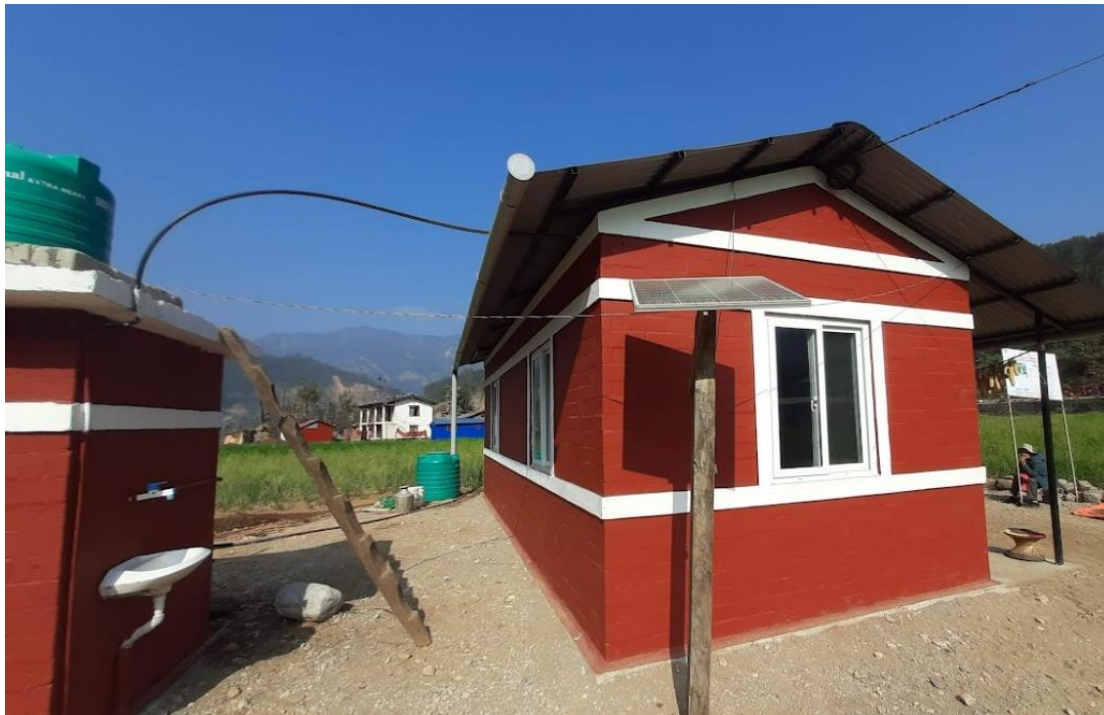
Figure 2 Post disaster reconstruction shelter (IOM model house) in Rimna, Jajarkot
