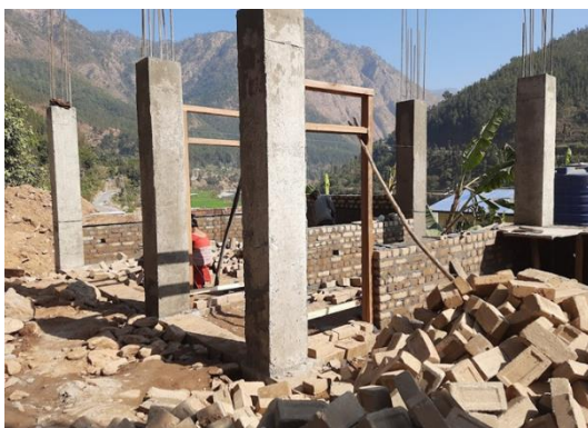
Figure 18 RCC building with CSEB brick under construction post disaster scenario
