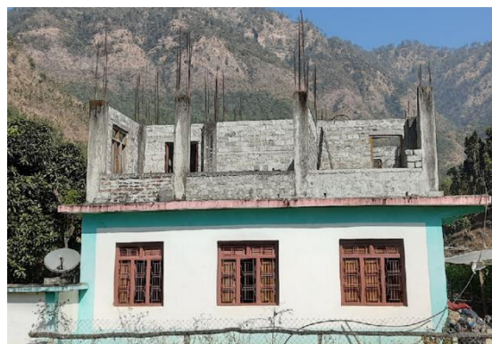
Figure 19 RCC building with cement block wall under construction post disaster scenario
