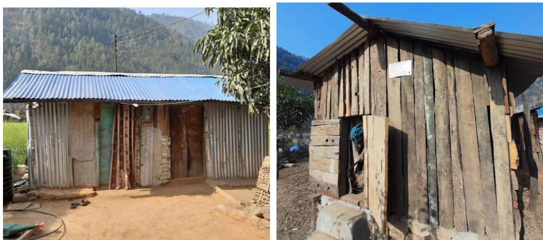
Figure 15 Temporary shelter constructed using CGI and reused materials from destroyed house in Rimna, Jajarkot
