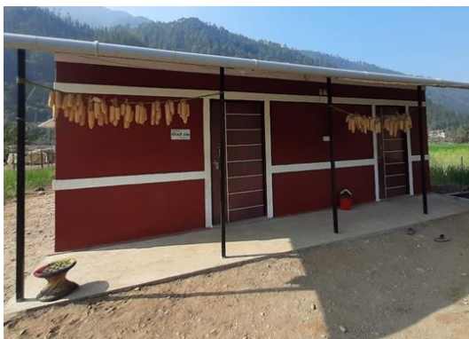
Figure 16 CSEB brick house constructed post disaster by IOM
