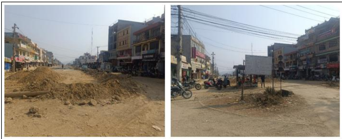
Figure 29 Under construction Road from Talchowk to Begnas Lake
