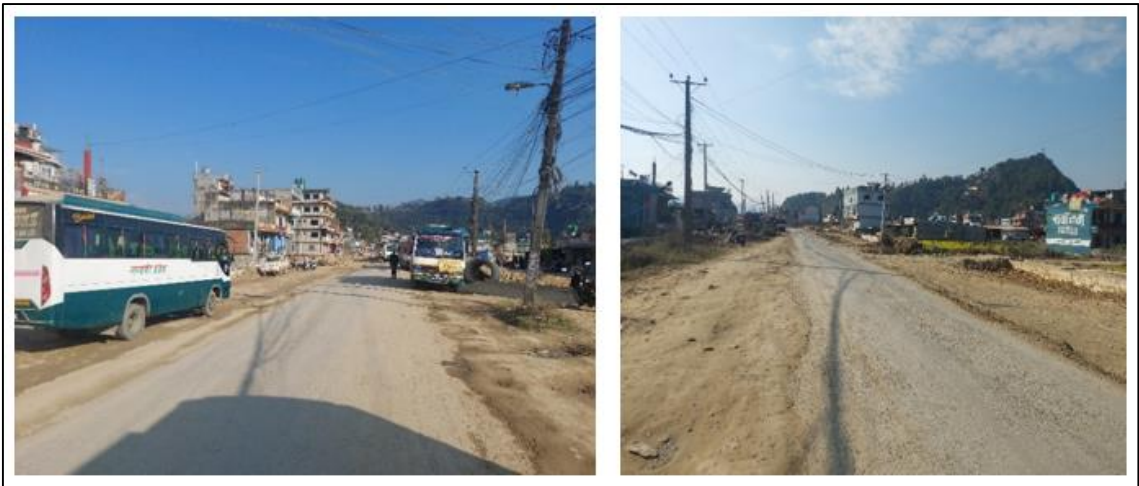
Figure 22 Begnas Bus Stop and Under Construction Road
