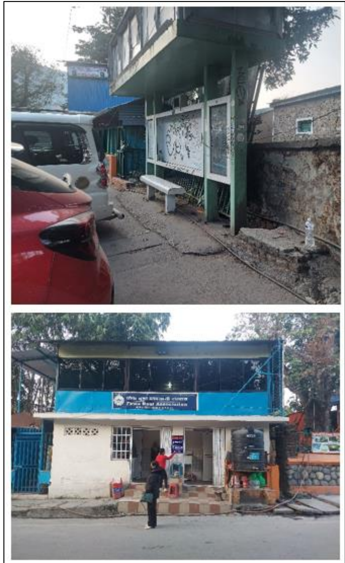
Figure 20 Public Toilet at Fewa Bus Stop
