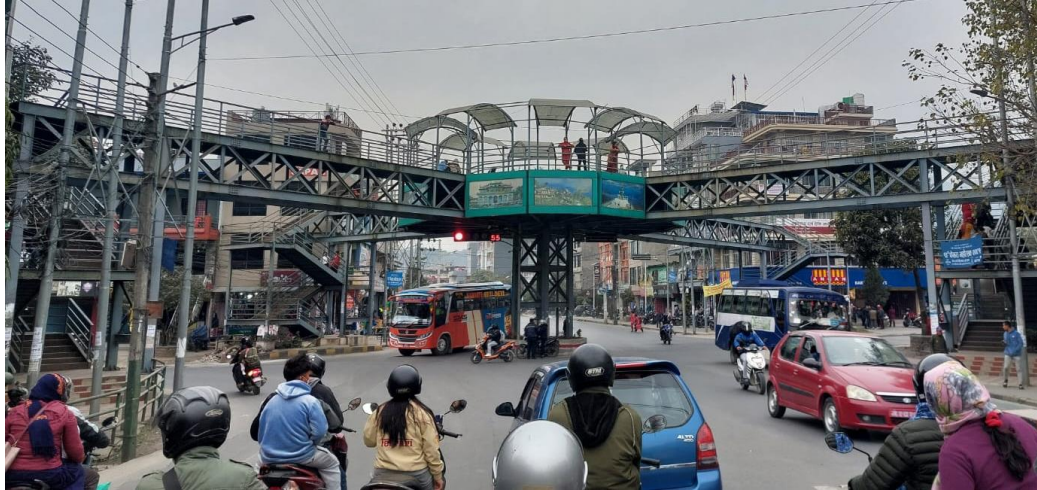
Figure 23 Traffic Signal at Srijanachowk
