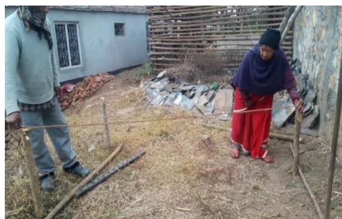
Image 5.4. Measuring Diagonals of Mat's Frame
