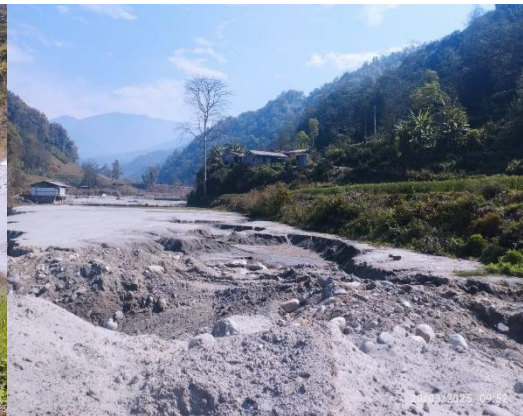
Figure 2 Indrawati III site
