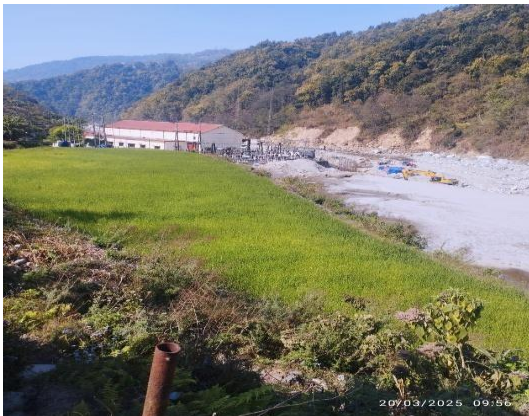
Figure 1 Indrawati III site
