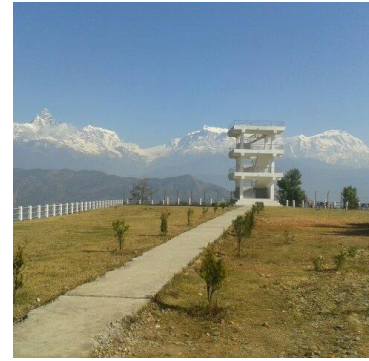
Figure 30 View tower located in place of shiva statue earlier.
