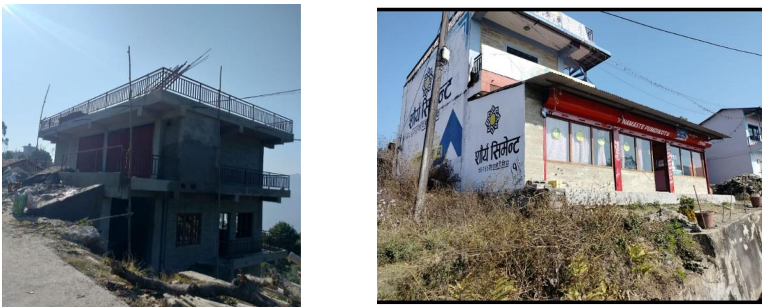
Figure 21 New houses with Shutters
