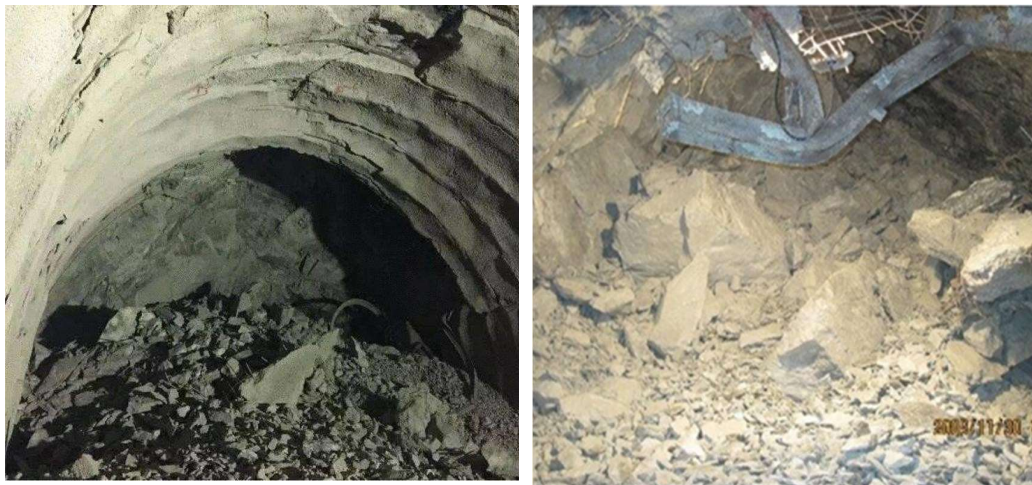
Figure 1.1: Rock burst (Source: Google)
