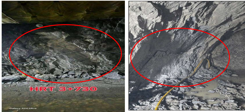
Figure 1.2: Rock burst (Rolwaling Khola Hydropower Project)
