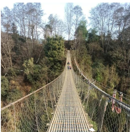
Figure 4.18: Bridge connecting Khopasi to Balthali
