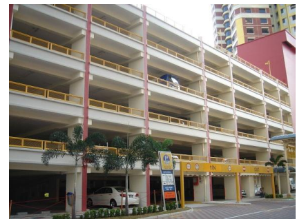
Figure 32: 3.24: Multi-storey carpark can be found at newer HDB estates in Singapore.
