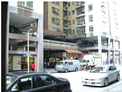
Figure 43: 3.35: Shops on ground and residence on floors above.
