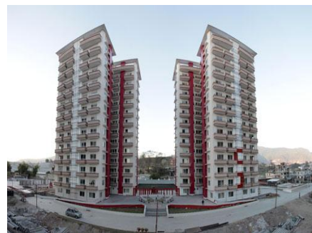
Figure 56: 3.48: High rise apartment
