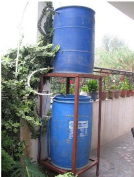
Fig.2-36: Treatment of water for Drinking- Bio Sand Filter (Shrestha R. R., Eco-Approach to Manage Wastewater, 2010)
