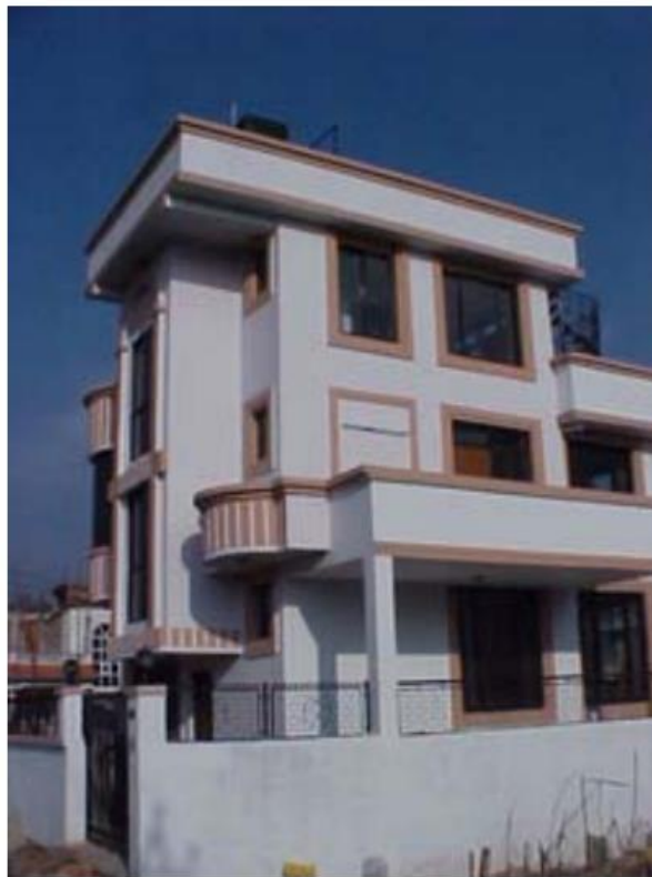
Fig.2-32: Eco home (Residence of Dr. Roshan Raj Shrestha)
