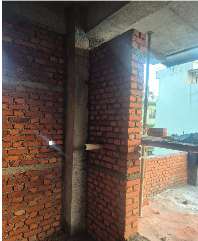
Photograph A7. 0.9 : Photograph at site S9
