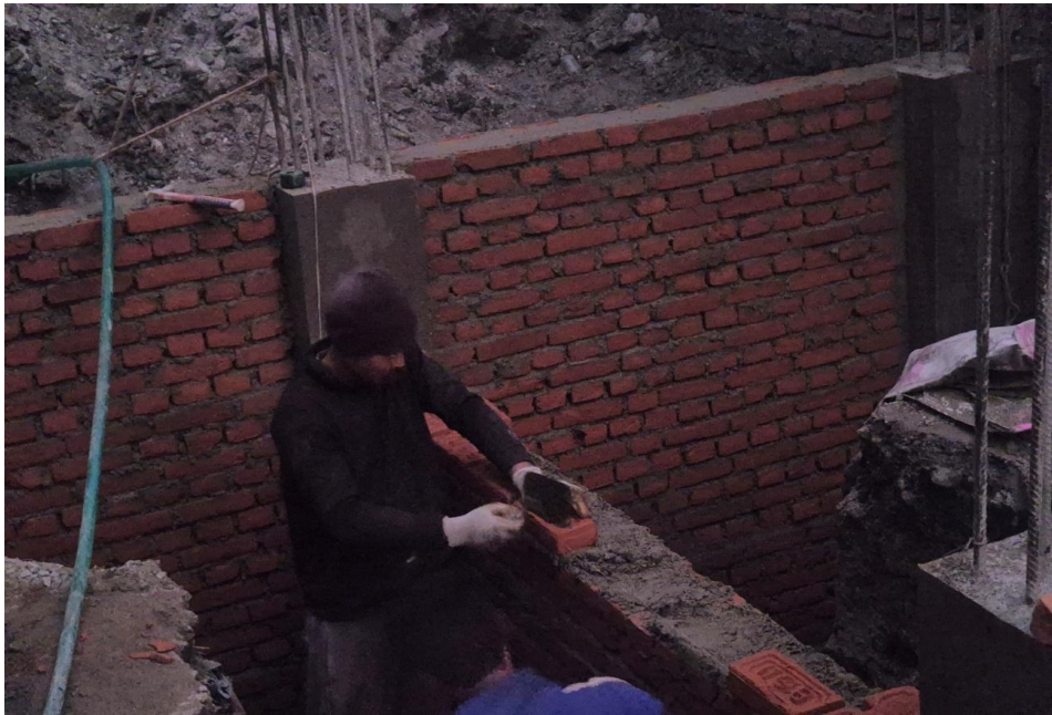
Photograph A7. 0.7 : Photograph at site S7
