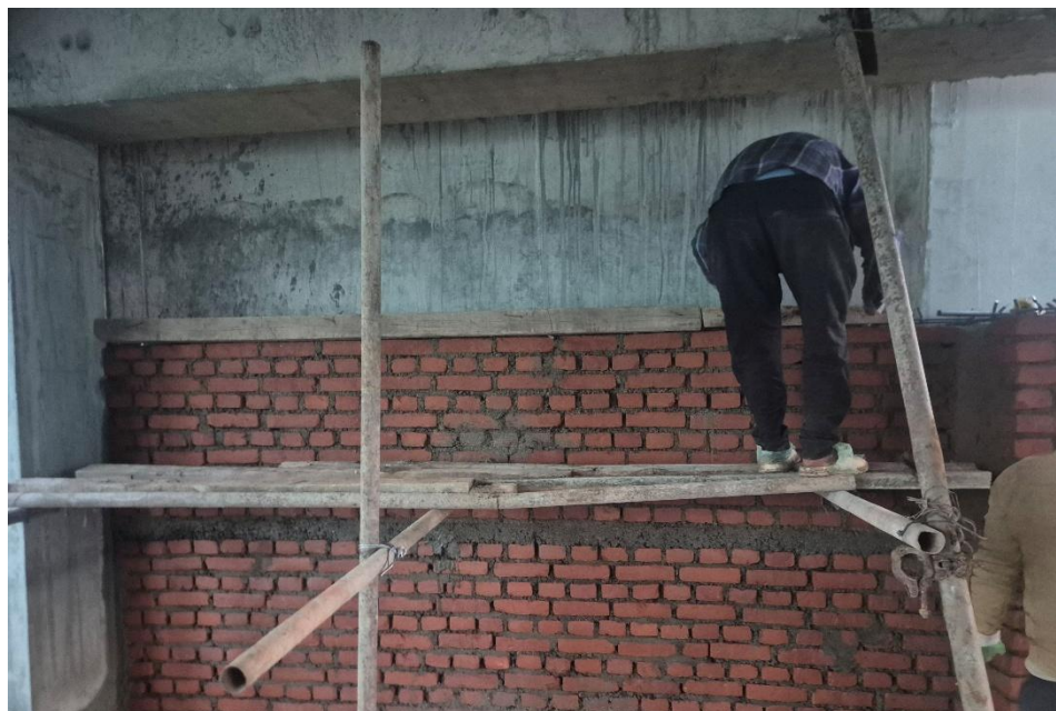
Photograph A7. 0.8: Photograph at site S8
