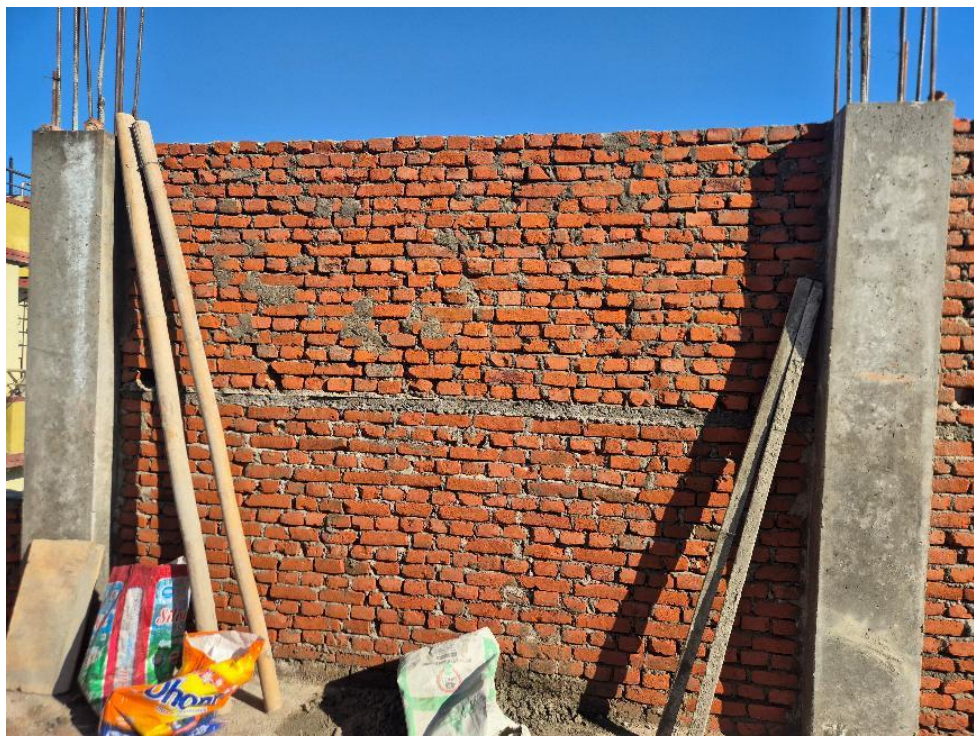
Photograph A7. 0.4: Photograph at site S4
