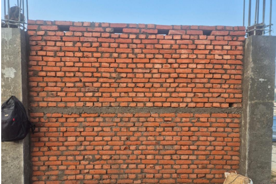
Photograph A7. 0.11 : Photograph at site S11
