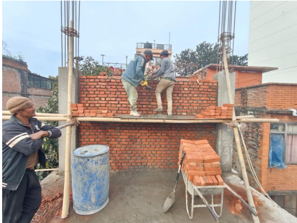
Photograph A7. 0.3 : Photograph at site S3
