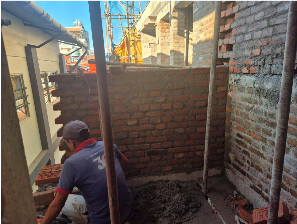
Photograph A7. 0.1: Photograph at site S1
