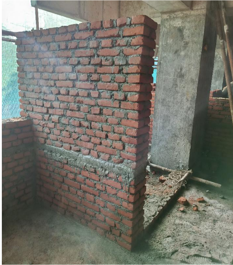
Photograph A7. 0.5: Photograph at site S5
