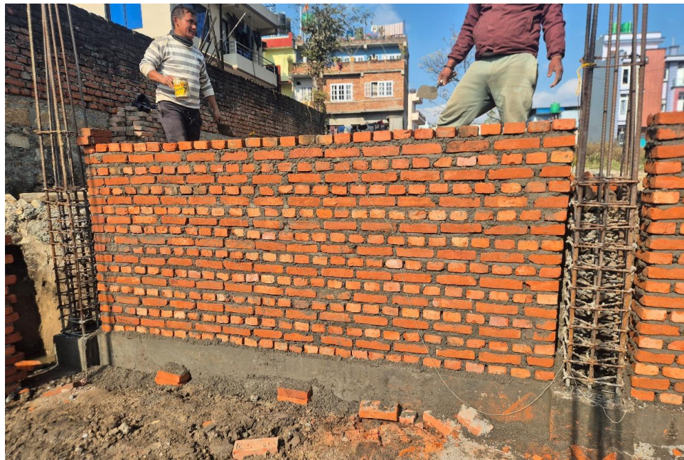
Photograph A7. 0.6: Photograph at site S6
