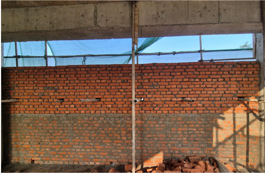
Photograph A7. 0.15 : Photograph at site S15
