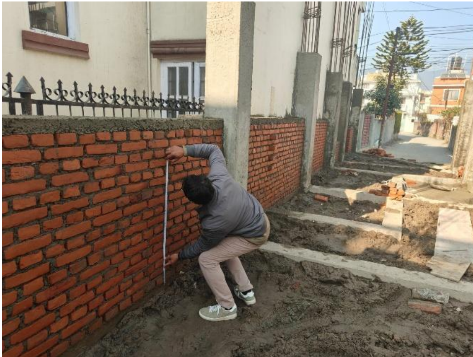
Photograph A7. 0.2: Photograph at site S2
