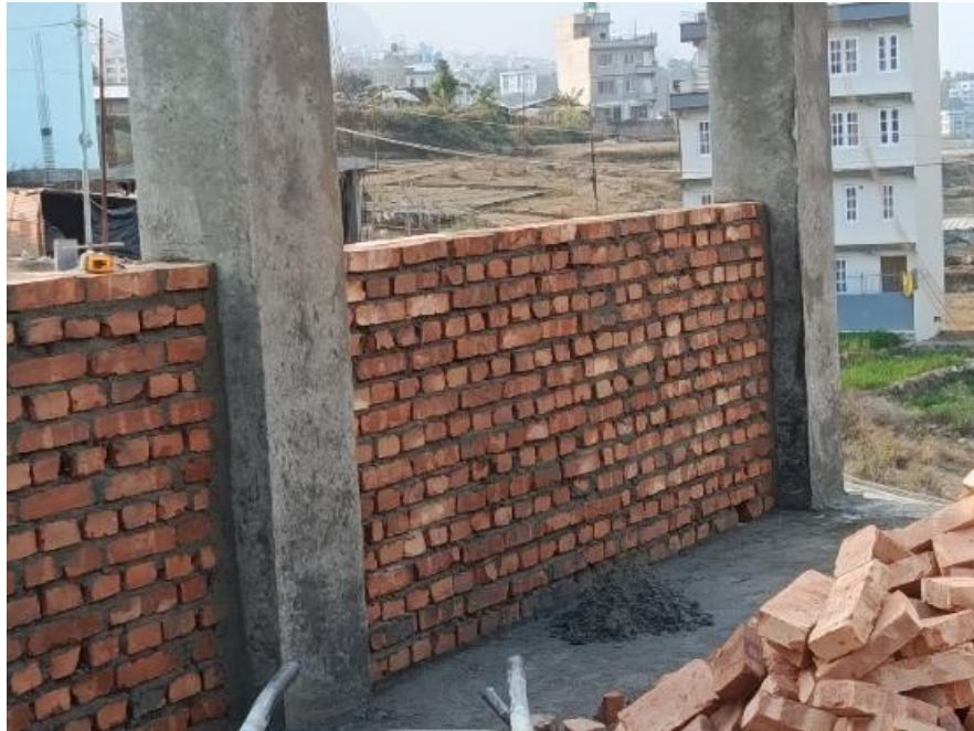
Photograph A7. 0.14 : Photograph at site S14
