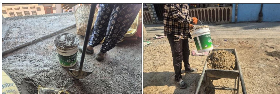
Photograph 3.2: Material measurement using standard box selected for study
