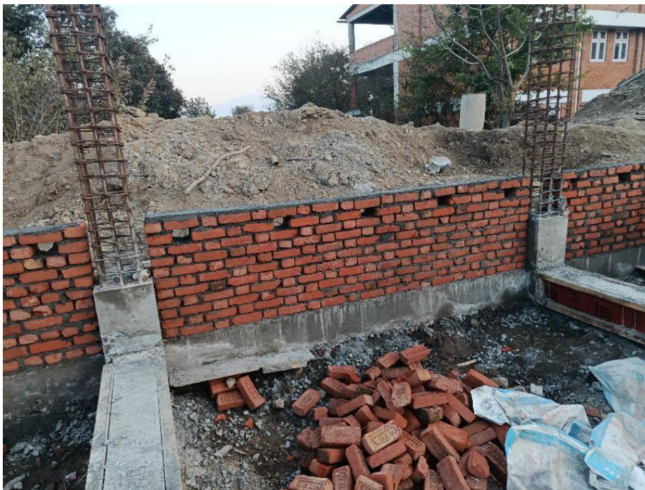
Photograph A7. 0.12 : Photograph at site S12
