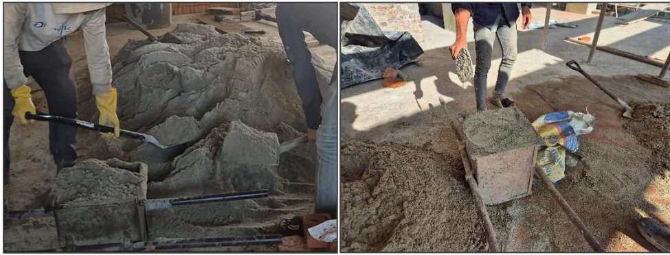
Photograph 3.3: Material measurement using standard box available on site
