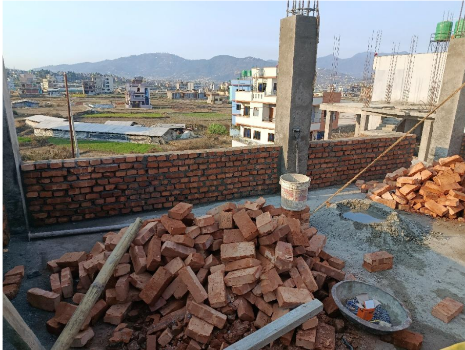
Photograph A7. 0.13 : Photograph at site S13
