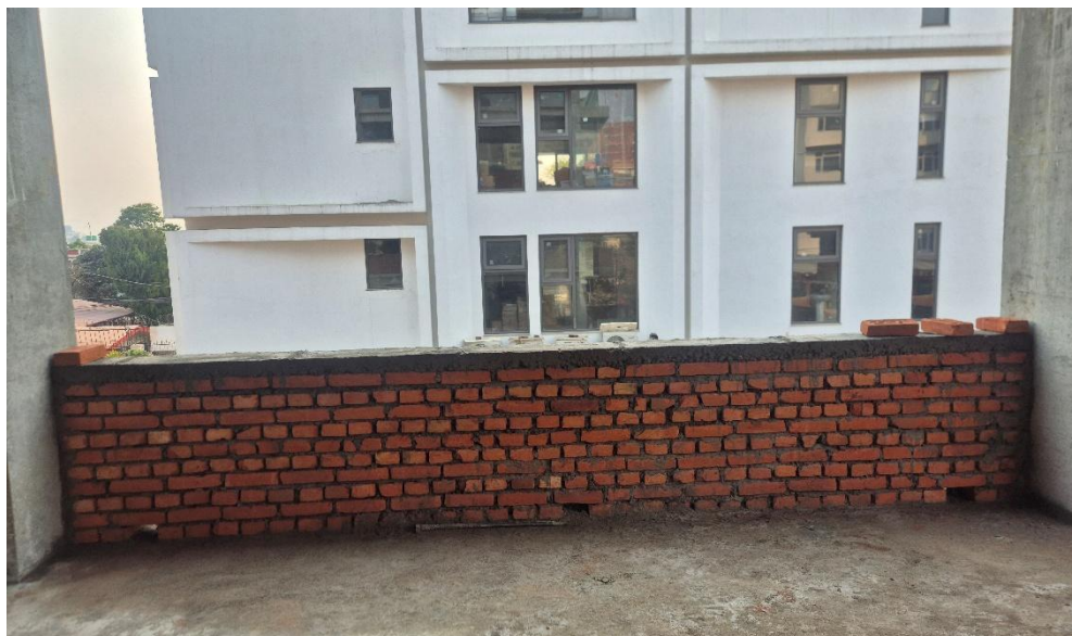
Photograph A7. 0.10 : Photograph at site S10
