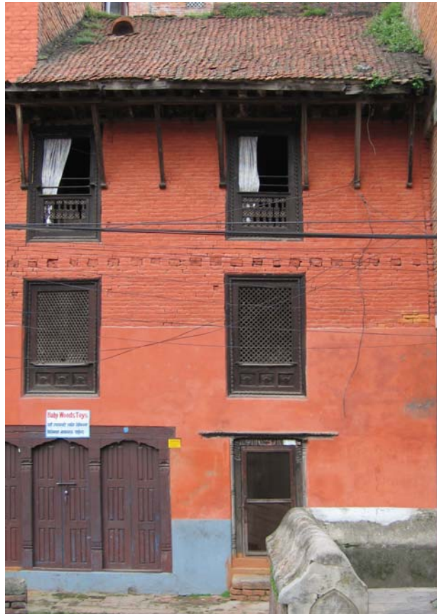
Figure 3.1: Traditional Masonry Dwelling House
