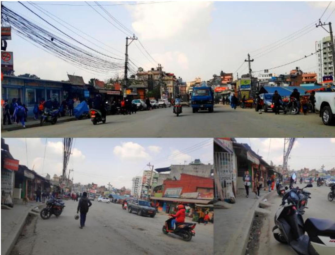
Figure 42 Road Towards Eantakuna Junction from Bottle neck Junction
