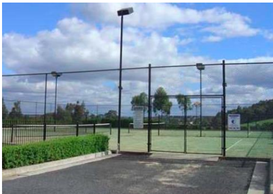
Figure 22 Tennis court, Macquarie Links
