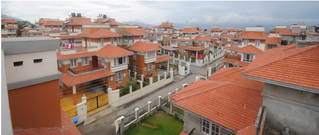
Figure 9 Civil Homes, Bhaishipati (The first housing colony in Kathmandu)
