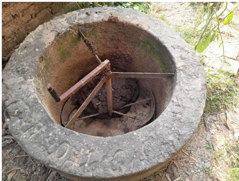
Figure B.6: Biogas Plant in Chitwan
