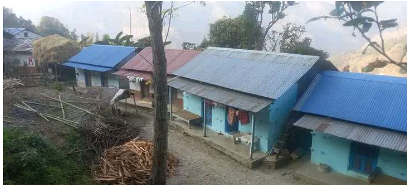
Figure B.1: Ramechhap Likhutamakoshi Houses
