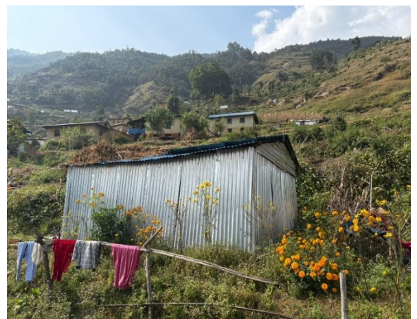
Temporary shelter in Barekot 3
