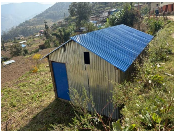
Temporary shelter in Barekot 2
