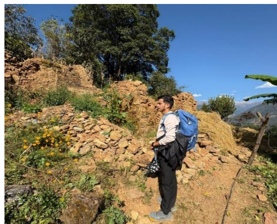
Researcher observing the damage caused
