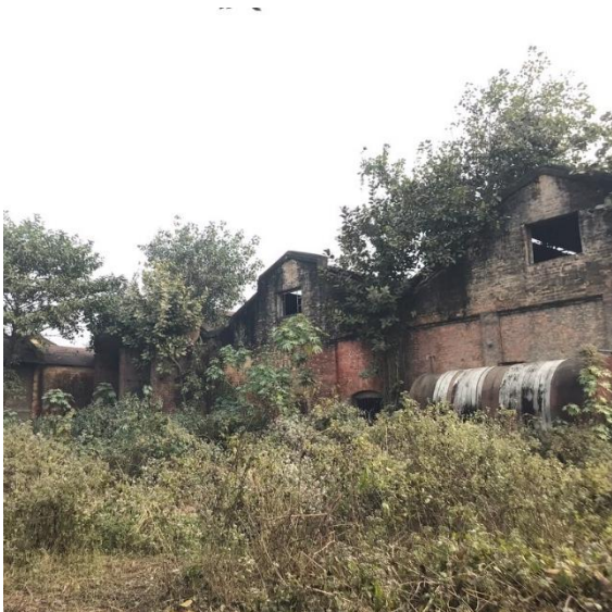
Figure 26 Jute Mills Main Building
