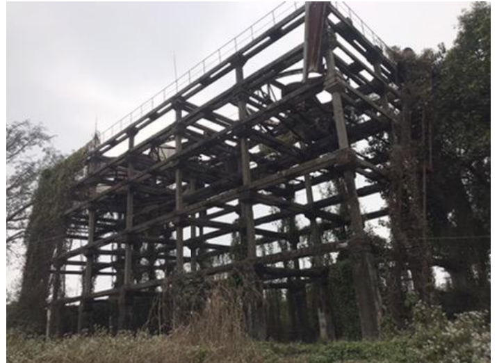
Figure 23 Structure to house crane
