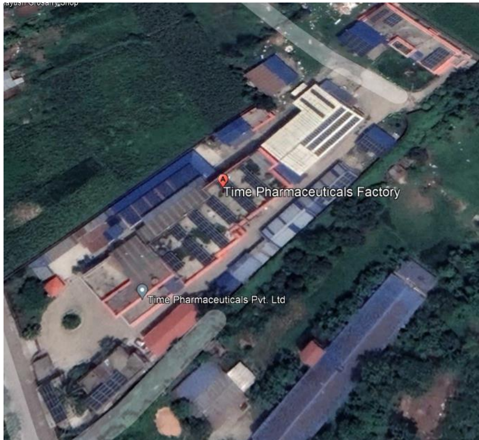
Figure 3.2: Google Earth map of solar PV plant installed in Time pharmaceutical factory
