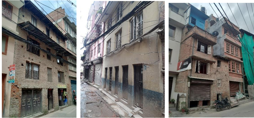
Figure 3.1 URM houses in urban areas with openings in Front Elevation
