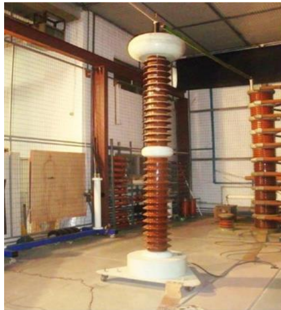
Figure 3.8: Load capacitor and external front resistor of the AUTH laboratory
