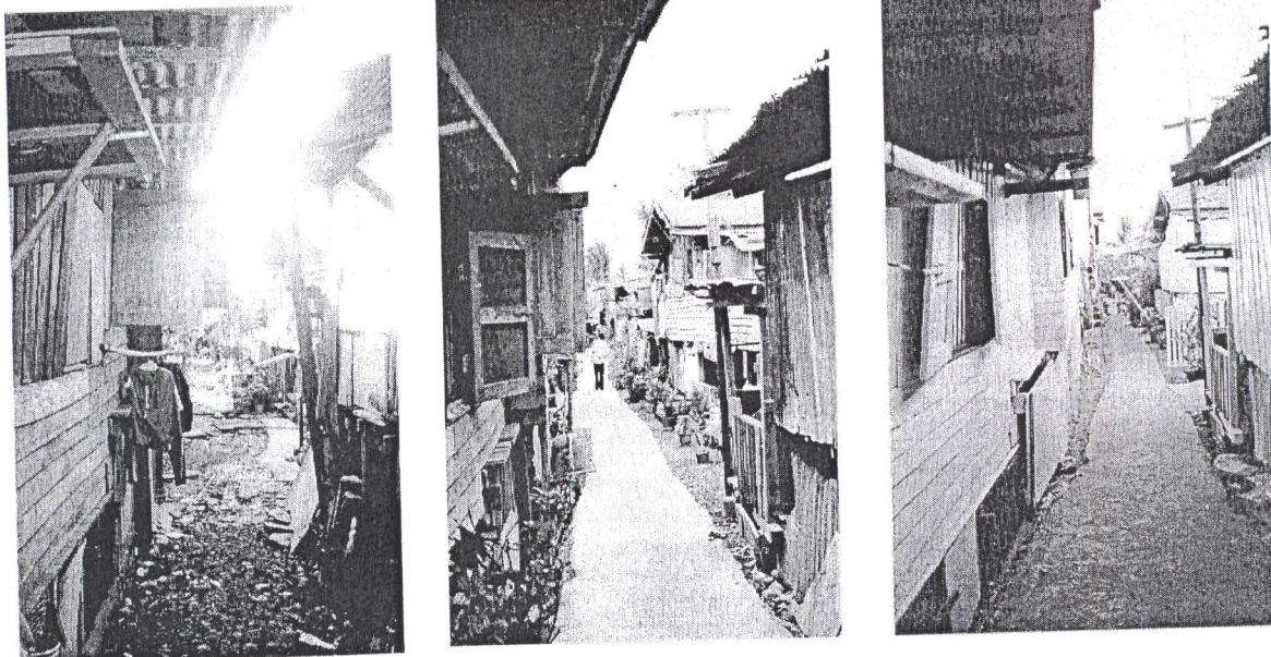
Fig 5.1: Showing the settlement before upgradation and after upgradation
