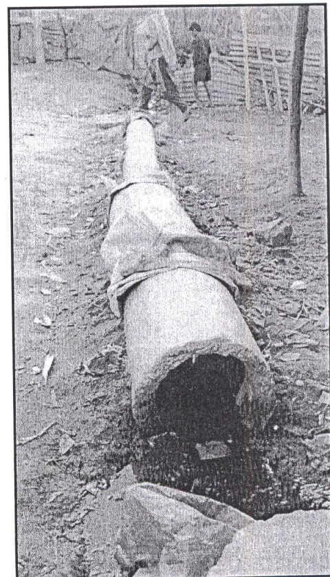
Fig:4.8 Side Drain
