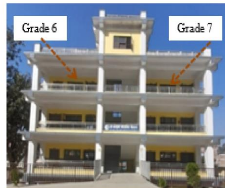
Figure 1: Case study building East facade showing the classroom used for study
